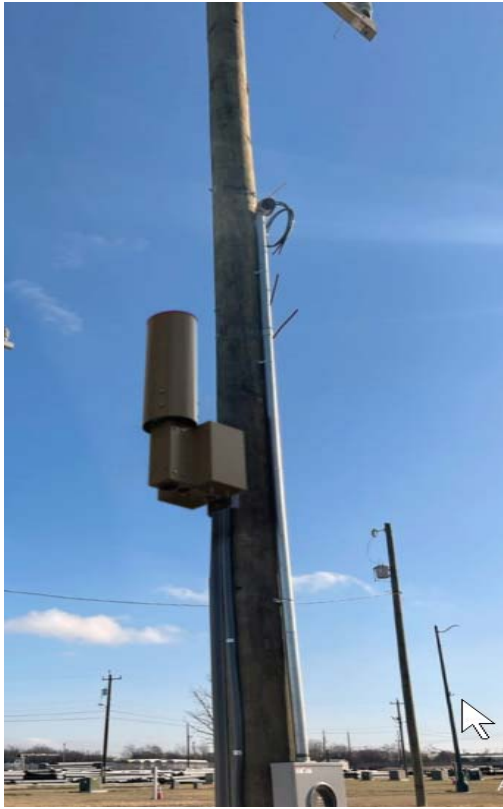
CPS Wood Pole "AFTER"
