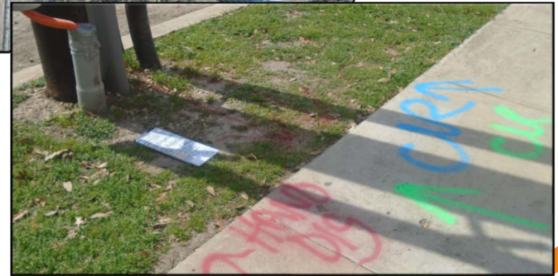
Locates on Sidewalk
