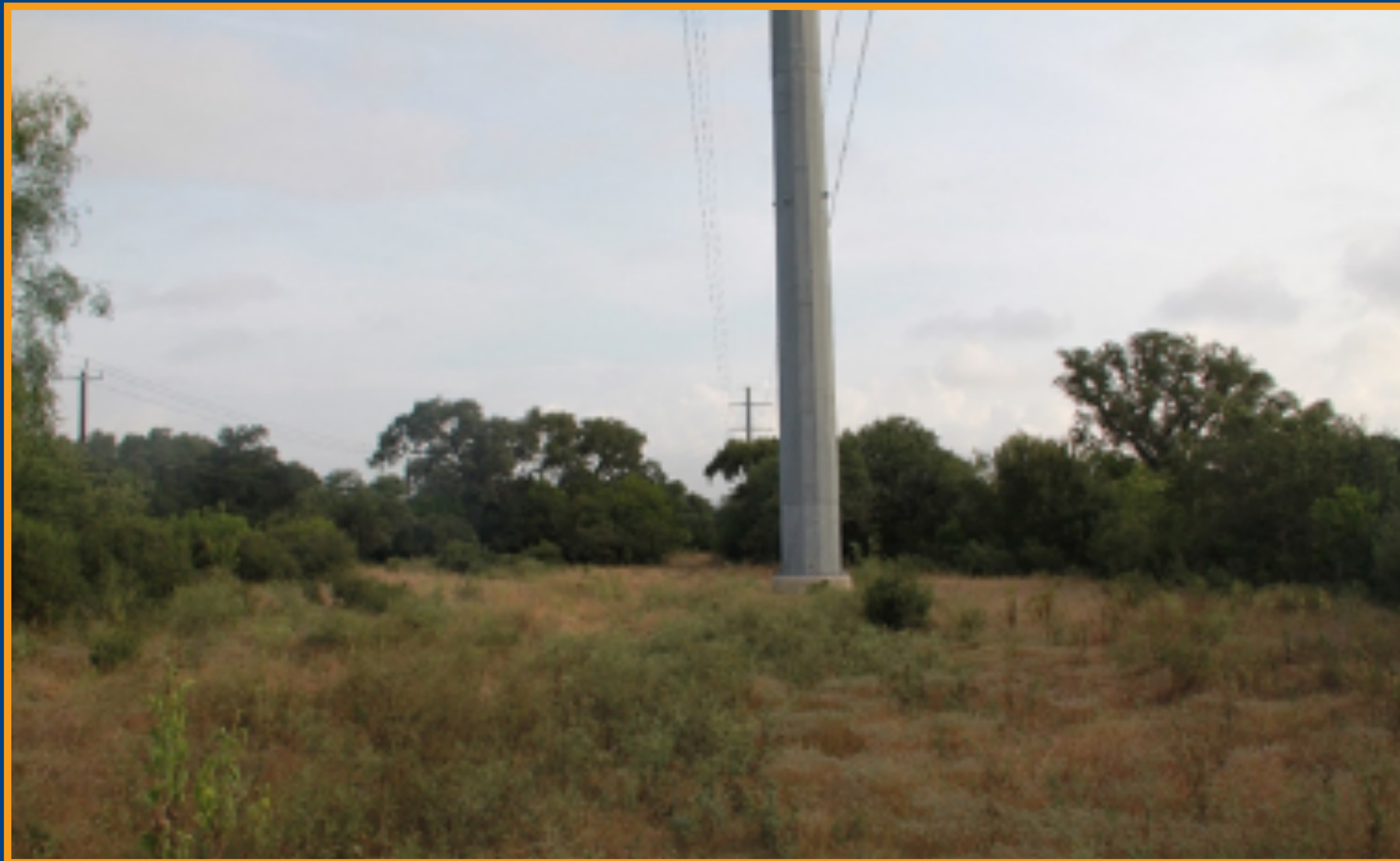
100 feet clearing around transmission structure
