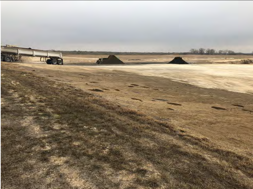
Photograph: 2 Fly Ash Landfill – standing on west berm – facing northeast. Photo taken 12/15/2020.
