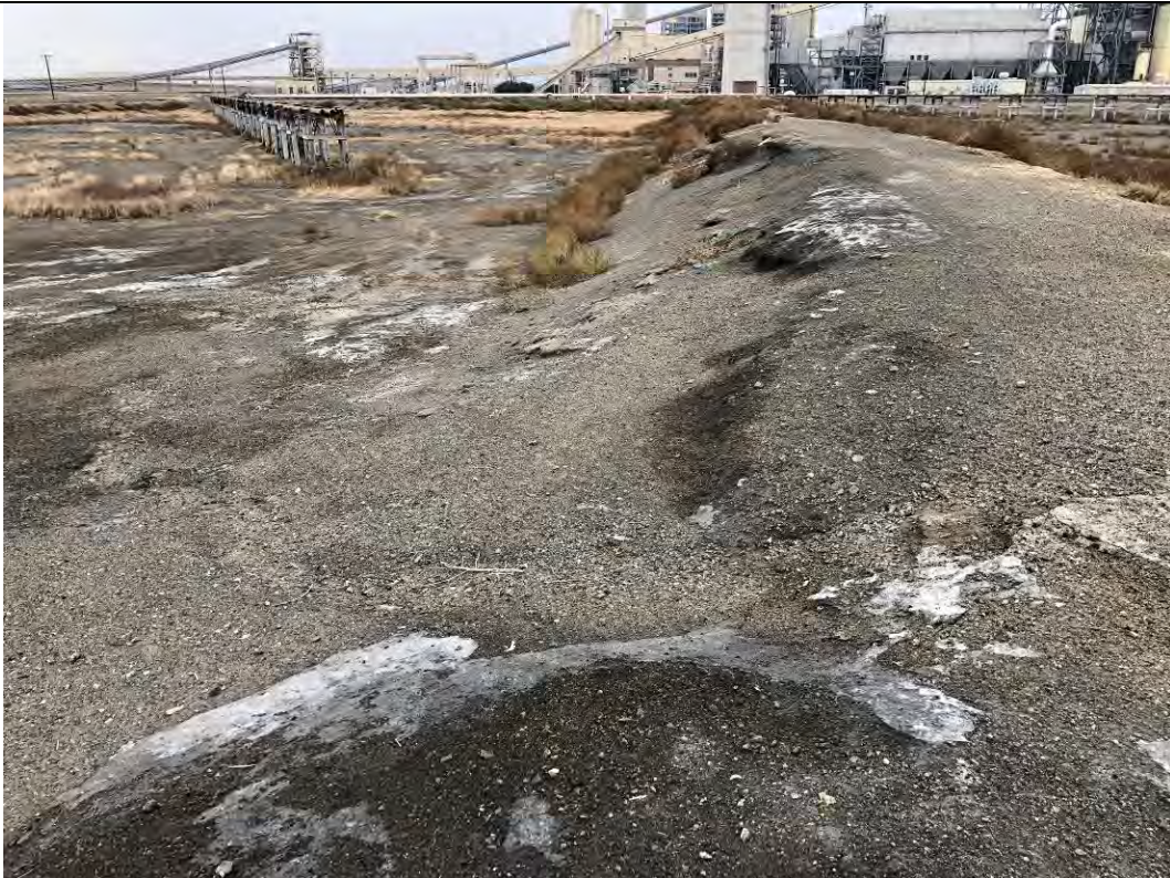
Photograph: 22 South Bottom Ash Pond – standing on northeast corner – facing west. Photo taken 12/15/2020.
