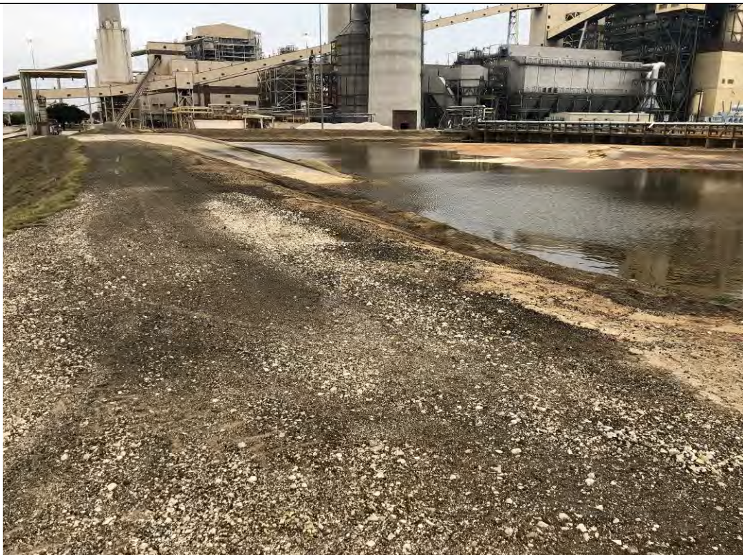
Photograph: 34 South SRH Pond – standing on the southeast corner – facing west. Photo taken 12/15/2020.
