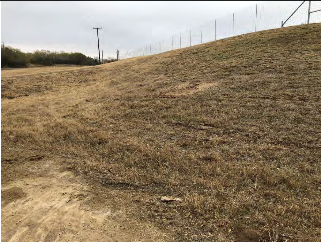
Photograph: 15 Evaporation Pond – standing on the southwest corner – facing north. Photo taken 12/15/2020.
