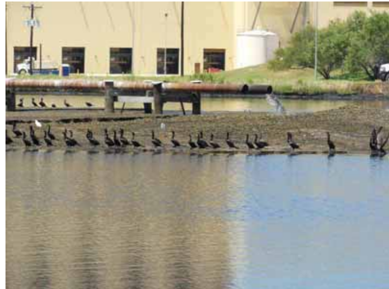
Photo 18: NP - Inlet piping, looking northwest. Piping includes one 8-inch diameter and two 12-inch-diameter pipes.
