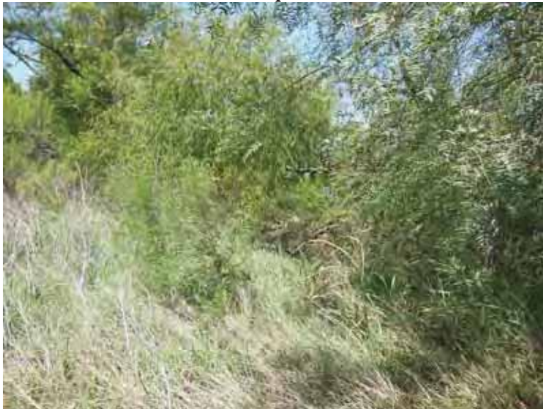
Photo 47: NP - Vegetation on north embankment exterior slope, looking north.
