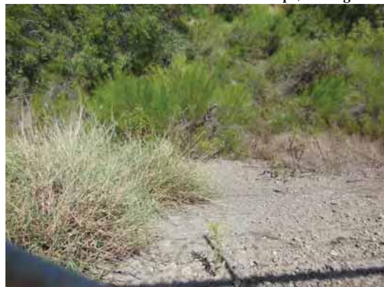
Photo 4: NP - North embankment exterior slope, looking north.
