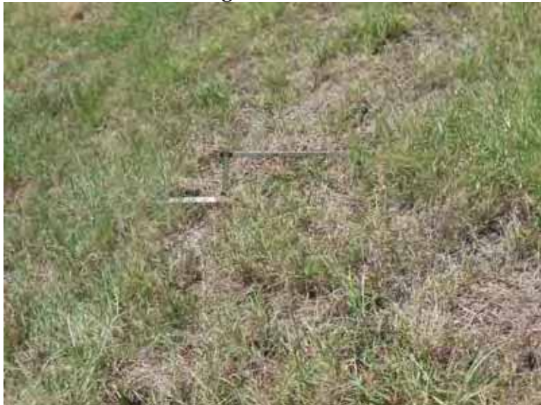
Photo 63: SP - Approximately 3H:1V side slope at south embankment exterior slope.
