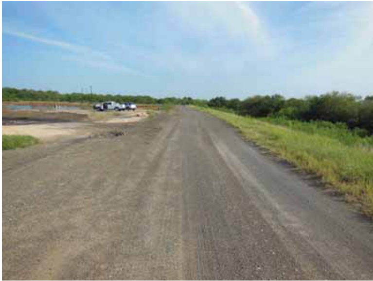
Photo 58: East Embankment crest, looking north.
