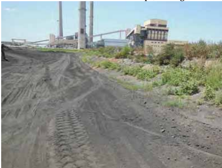
Photo 55: NP/SP - Common embankment south slope, looking west.
