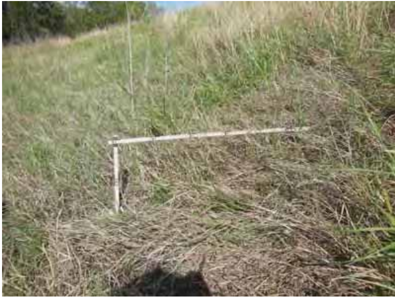
Photo 118: South embankment exterior slope measured approximately 3H:1V.
