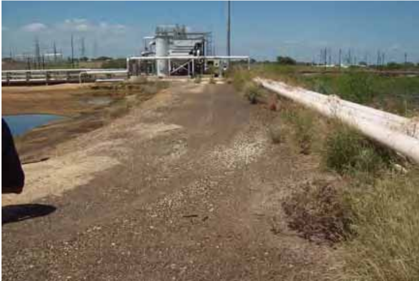
Photo 73: SP - West embankment crest, looking north.
