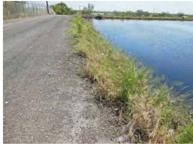
Photo 6: NP - North embankment interior slope, looking east.
