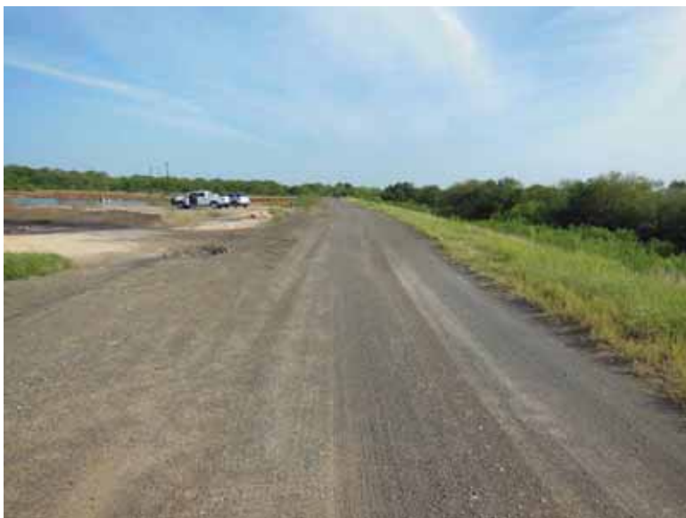
Photo 90: East Embankment crest, looking north.
