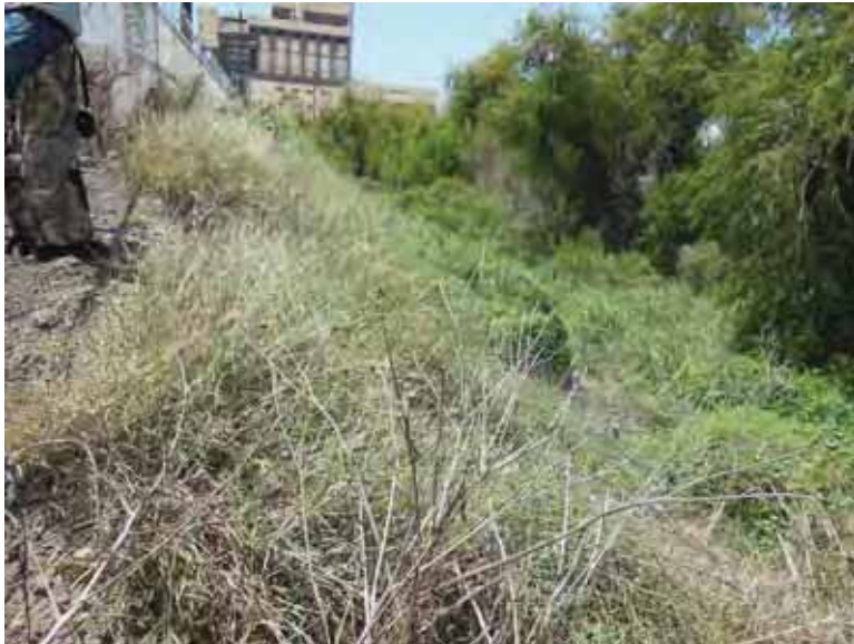
Photo 49: NP - North embankment exterior slope, looking west.
