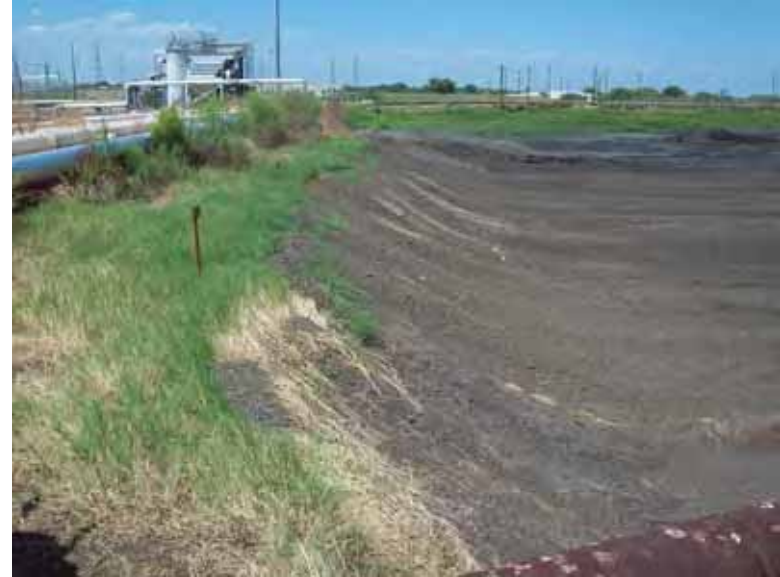
Photo 70: SP - West embankment interior slope, looking north.
