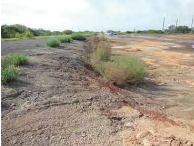
Photo 102: East embankment interior slope, looking south.
