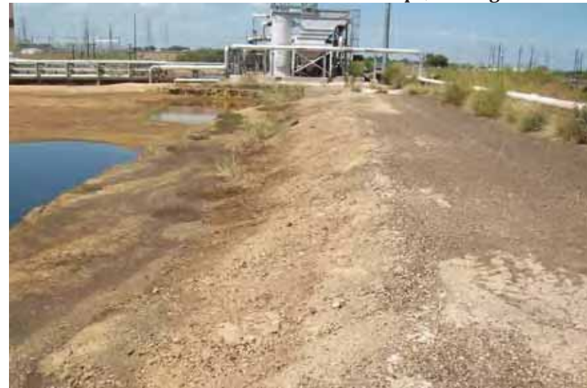
Photo 4: East embankment interior slope, looking north.
