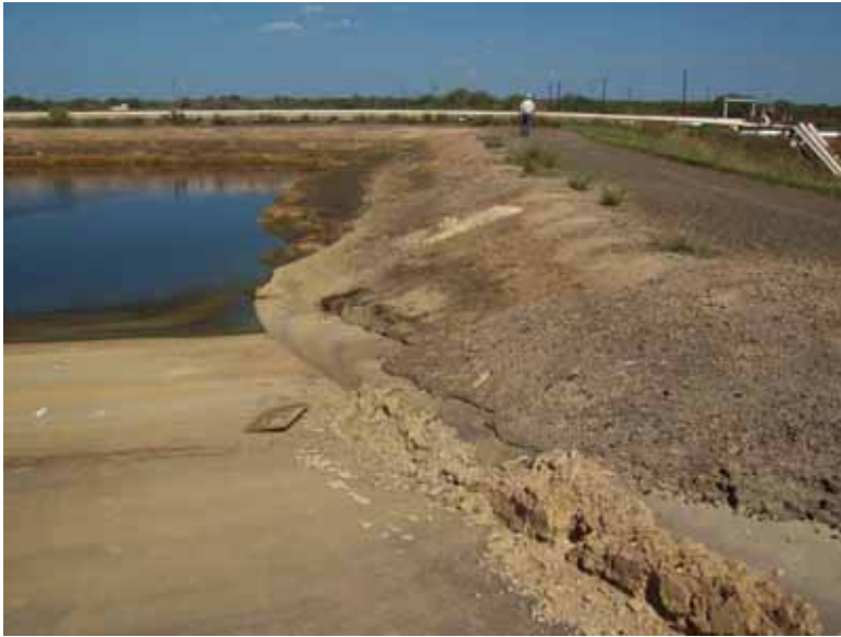
Photo 53: South embankment interior slope, looking east.
