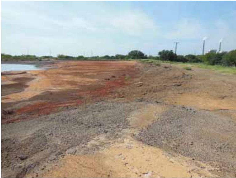
Photo 74: West embankment interior slope, looking south.
