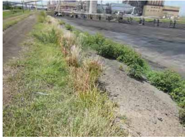
Photo 66: SP – South embankment interior slope, looking west.
