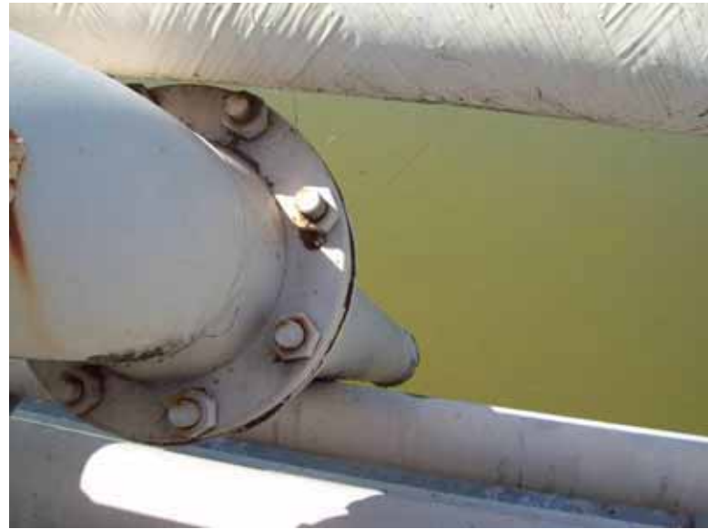
Photo 42: 6-inch-diameter metal SRH-north inlet pipe labeled "Waste Slurry Sump", looking north.
