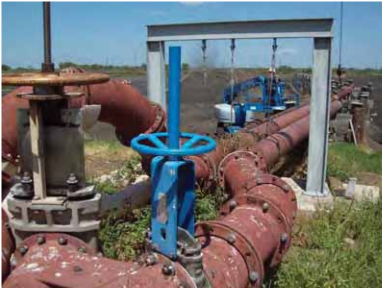
Photo 71: SP - Inlet piping at southwest corner interior slope, looking northeast.
