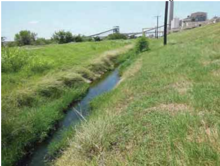
Photo 67: SP - Drainage ditch at south embankment exterior toe, looking west.
