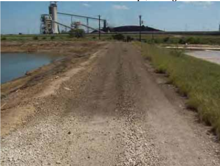
Photo 47: West embankment crest, looking south.
