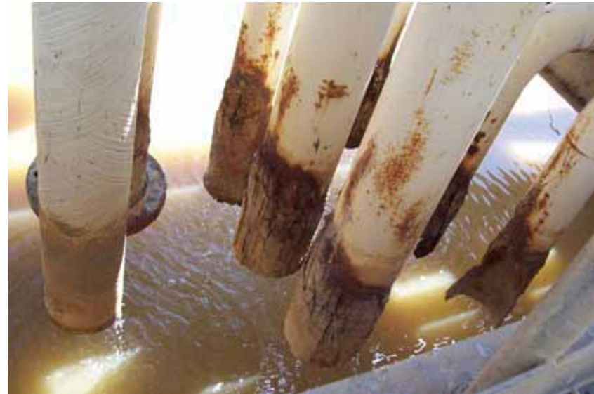
Photo 34: Nine outlet pipes into SRH-south, looking south.
