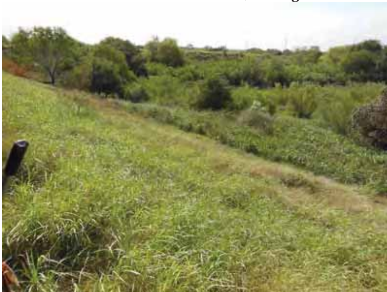
Photo 116: South embankment exterior slope, looking southeast.
