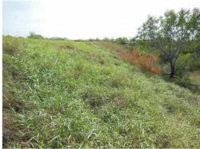
Photo 87: South embankment exterior slope, looking east.
