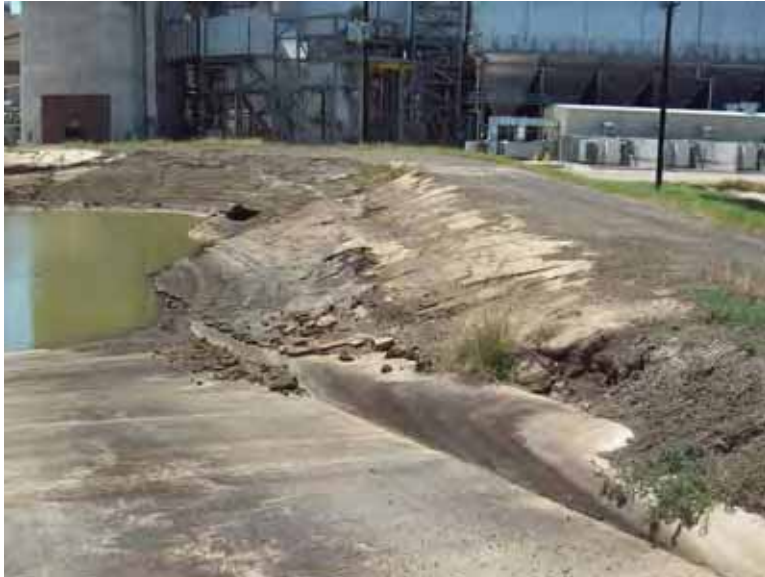
Photo 17: North embankment interior slope, looking west.
