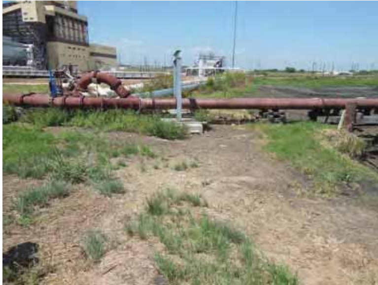
Photo 69: SP - Inlet piping at southwest corner interior slope, looking north.
