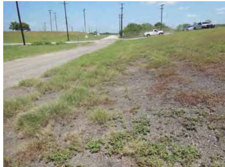
Photo 44: NP - West embankment exterior slope, looking north.
