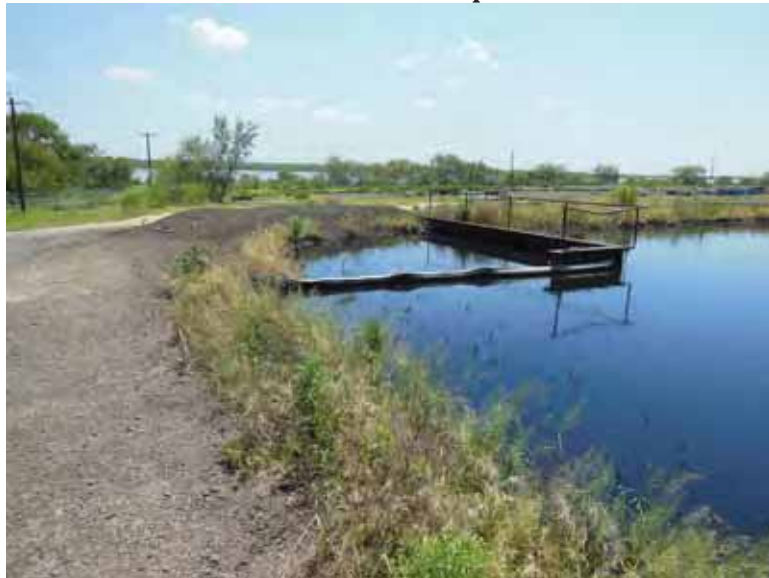
Photo 7: NP - Outlet structure at northeast corner, looking east.
