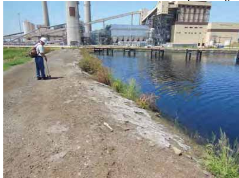
Photo 32: NP/SP - Common embankment north slope, looking west.
