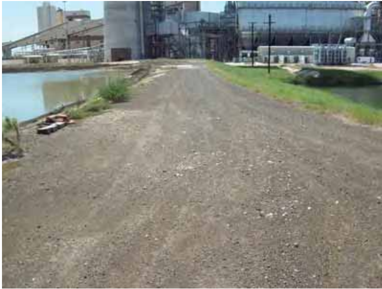
Photo 13: North embankment crest, looking west.
