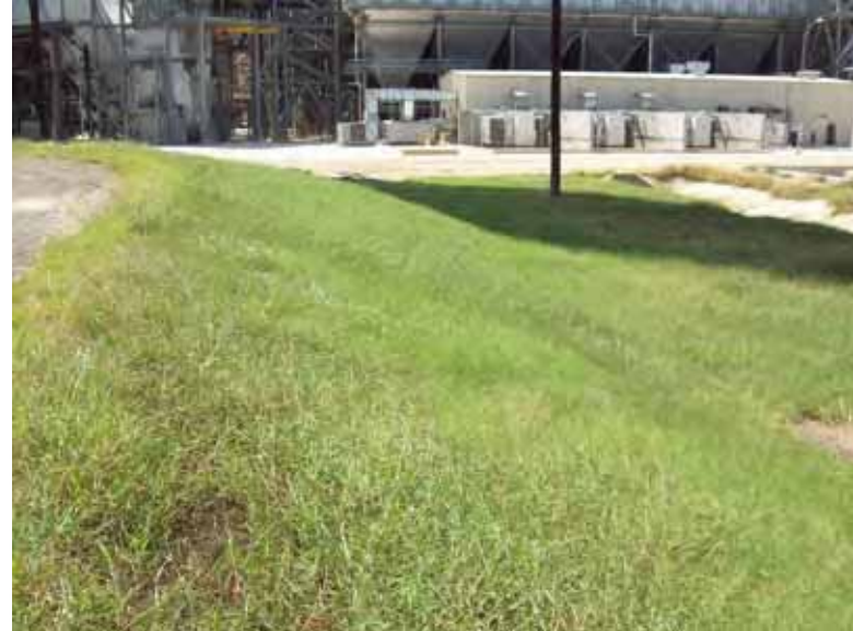
Photo 18: North embankment exterior slope, looking west.
