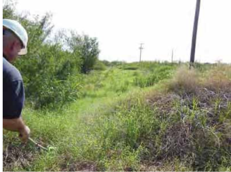
Photo 103: North embankment exterior slope, looking east.
