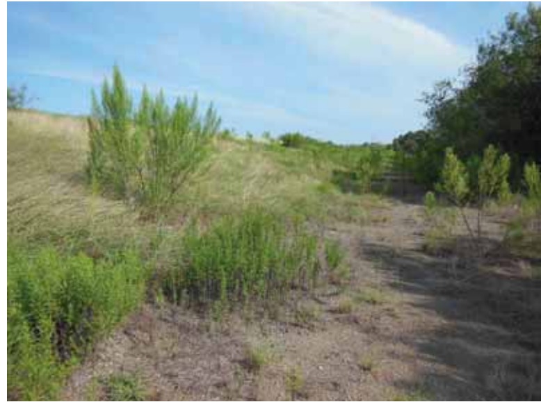
Photo 95: East embankment exterior toe, looking north.
