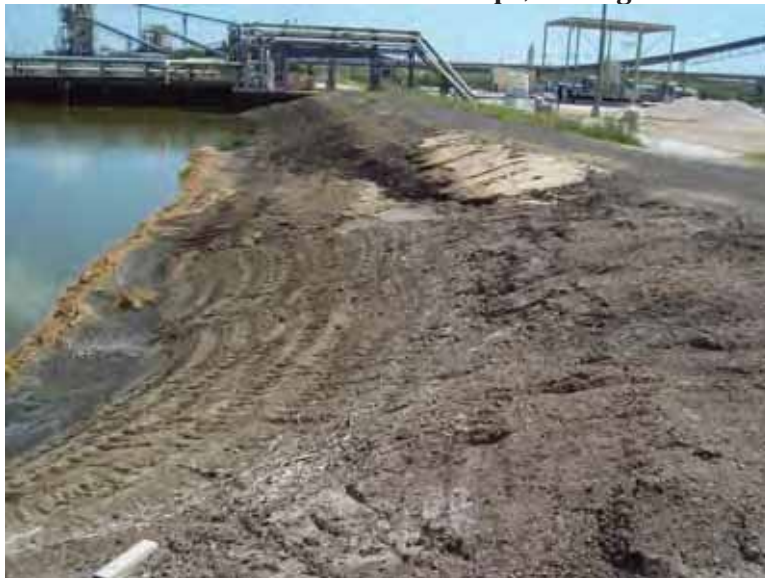
Photo 19: West embankment interior slope, looking south.
