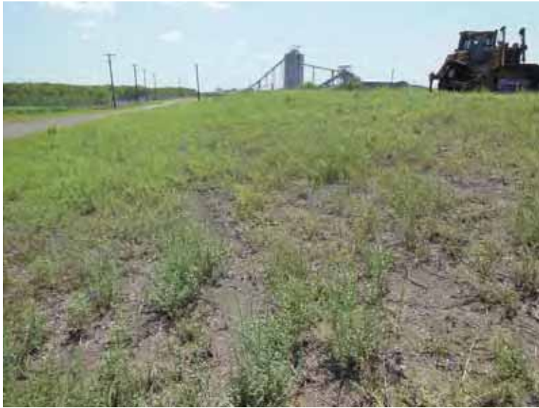
Photo 53: SP - East embankment exterior slope, looking south.
