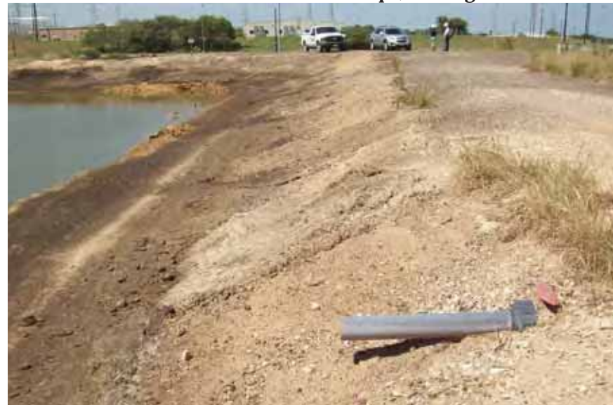
Photo 12: East embankment interior slope, looking north.
