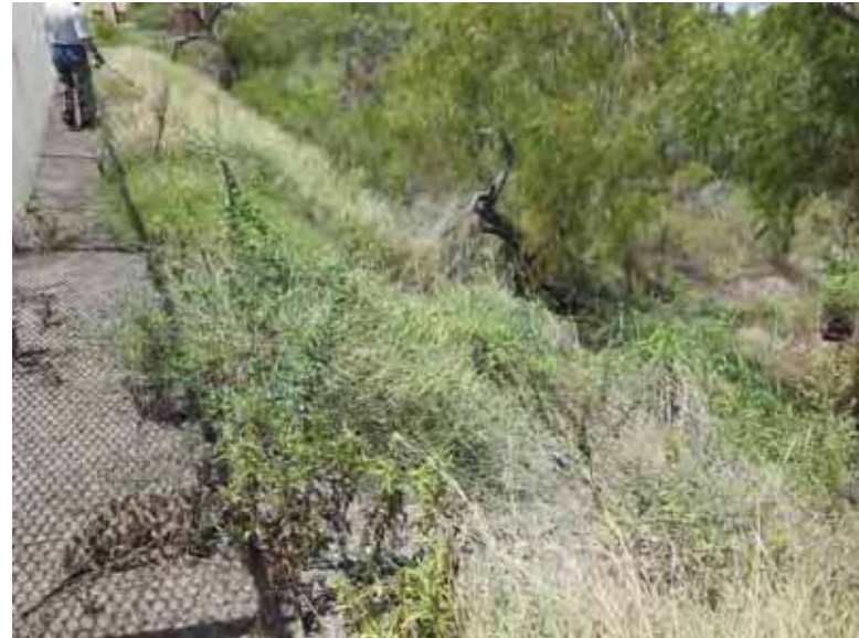
Photo 50: NP - North embankment exterior slope, looking west.
