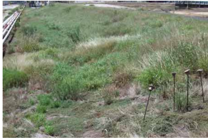
Photo 2: South embankment exterior slope, looking west.
