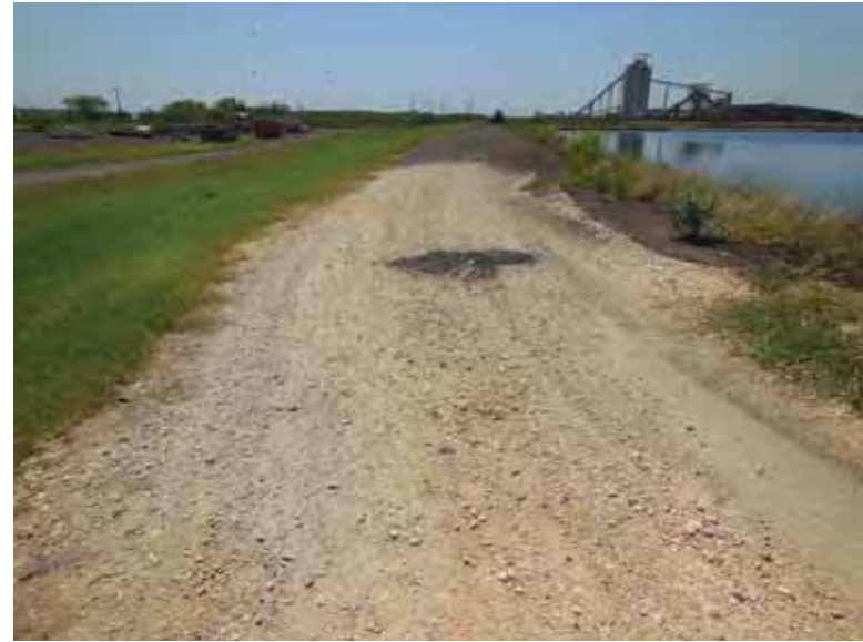
Photo 10: NP - East embankment crest, looking south.
