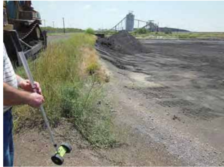
Photo 54: SP - East embankment interior slope, looking south.
