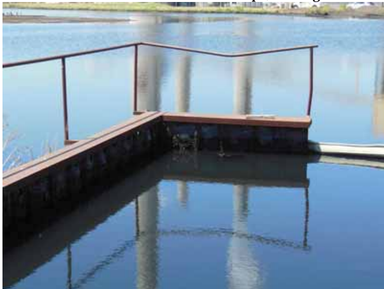
Photo 11: NP - Outlet structure at northeast corner, looking west. Outlet riser pipe.
