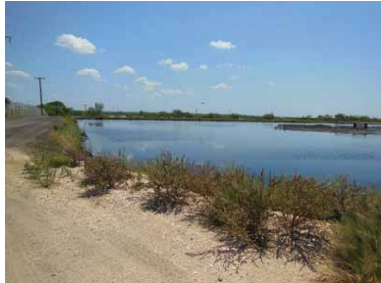
Photo 2: NP- North embankment interior slope, looking east.
