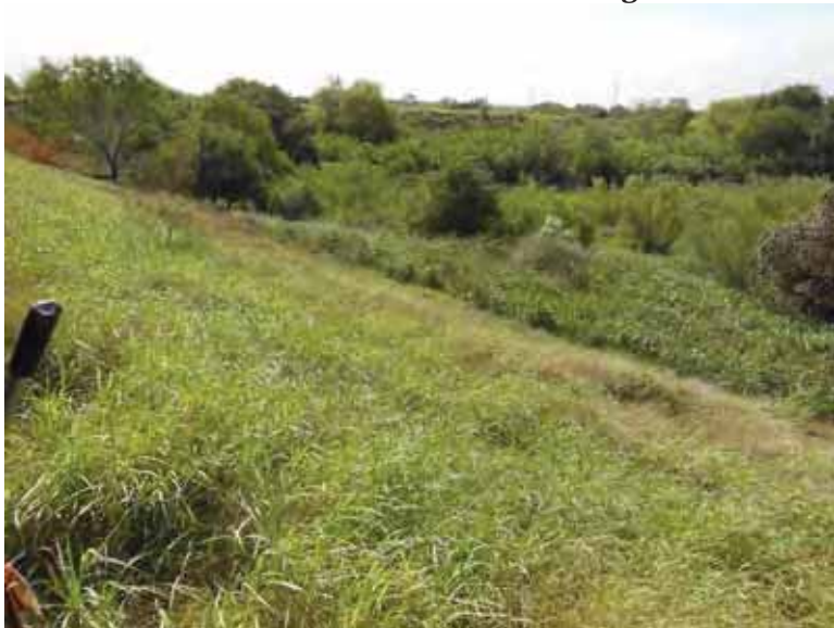
Photo 84: South embankment exterior slope, looking southeast.
