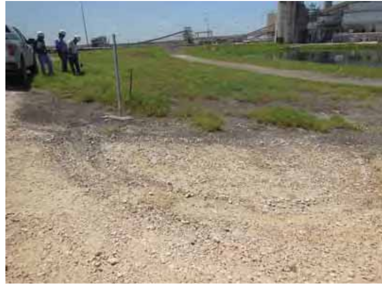
Photo 46: NP - Northwest corner exterior slope, looking south.
