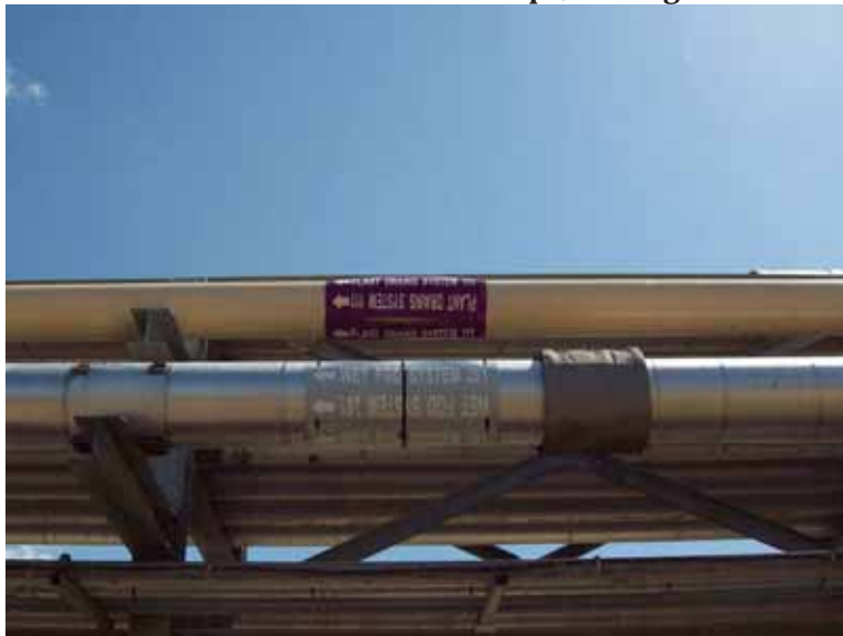
Photo 23: Overhead piping at west embankment crest, looking south.
