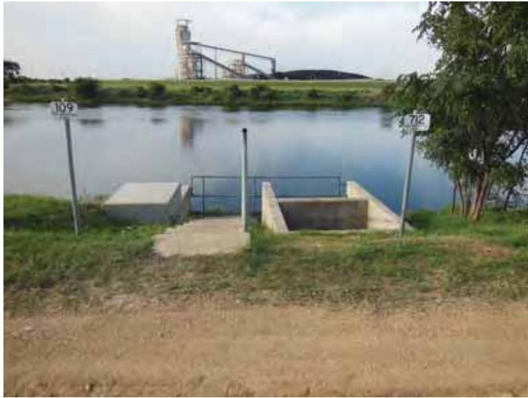
Photo 57: SRH outfall 109, looking south.
