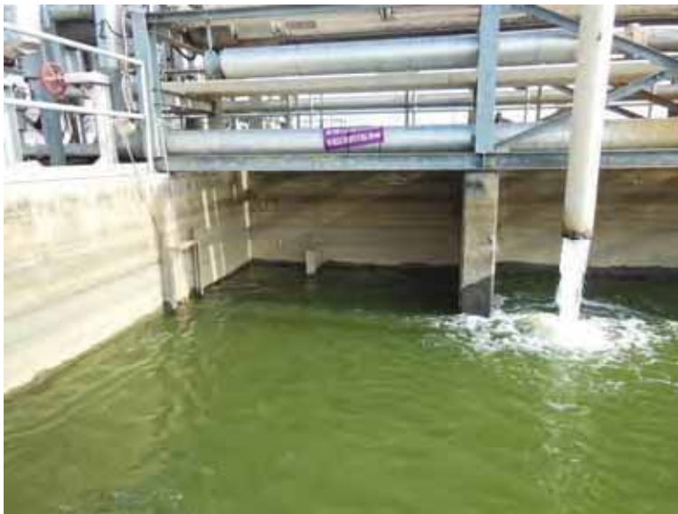
Photo 27: Submerged SRH-south outlet structure at west embankment interior slope, looking north.
