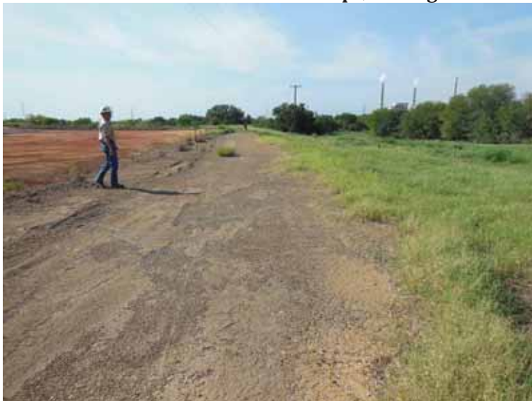
Photo 108: West embankment crest, looking south.
