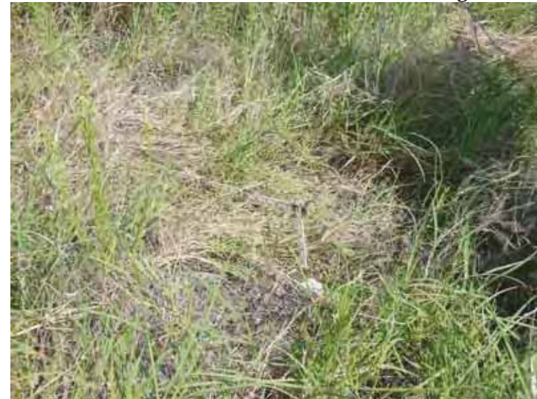
Photo 97: East embankment exterior slope measured approximately 4H:1V.
