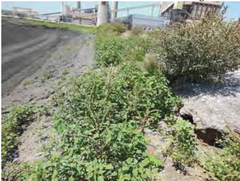
Photo 31: NP/SP - Common embankment south slope, looking west.
