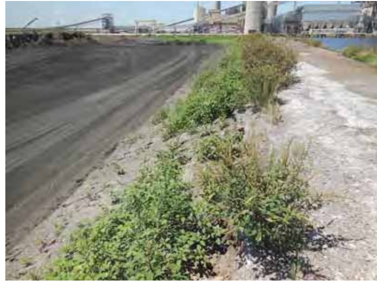
Photo 30: NP/SP - Common embankment south slope, looking west.
