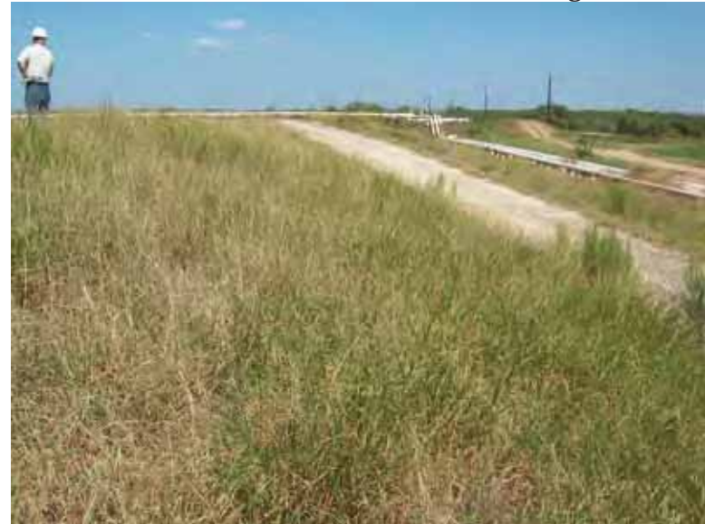
Photo 52: South embankment exterior slope, looking east.
