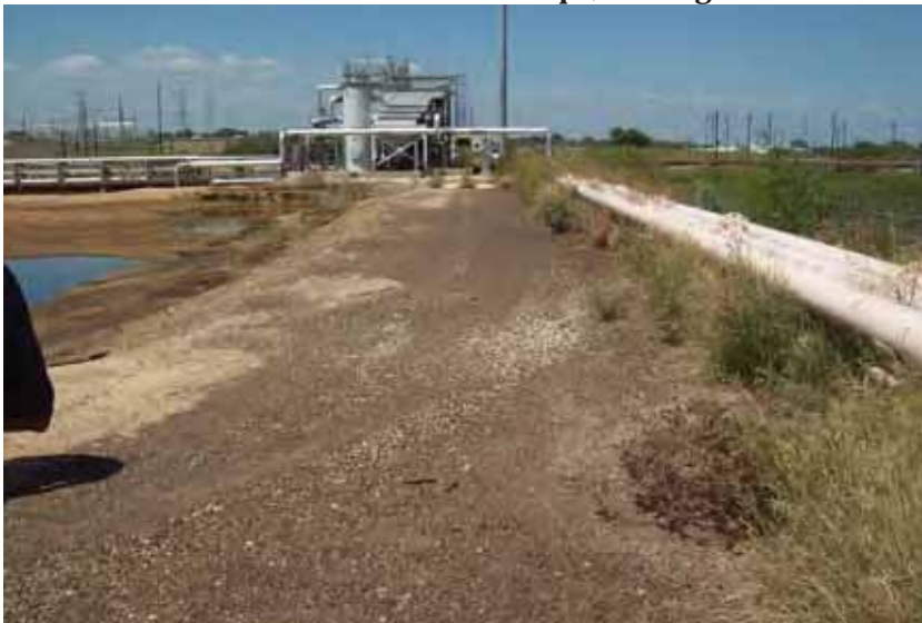
Photo 3: East embankment crest, looking north.
