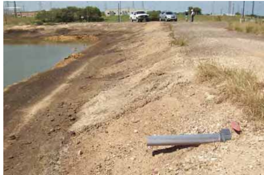
Photo 82: SP - West embankment exterior slope, looking north.
