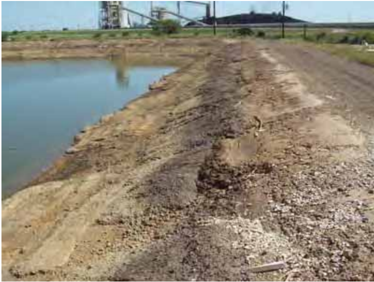
Photo 45: West embankment interior slope, looking south.
