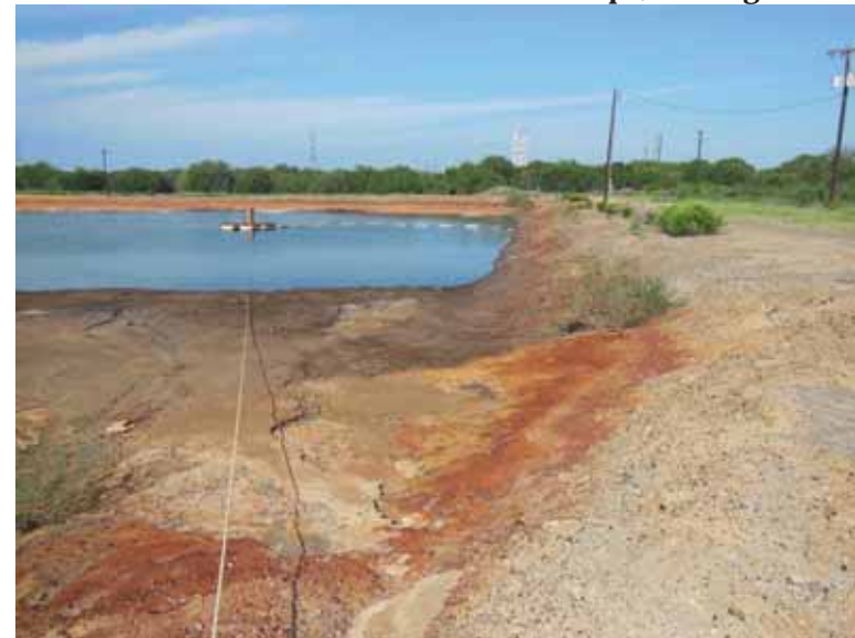
Photo 69: North embankment interior slope, looking west.
