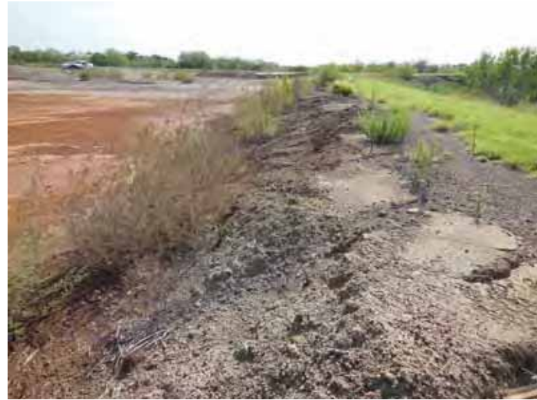
Photo 83: South embankment interior slope, looking east.
