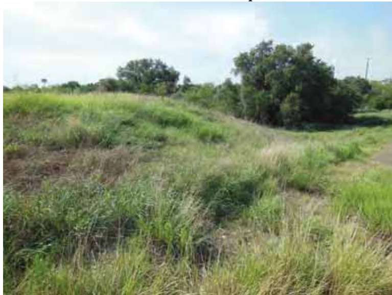
Photo 80: West embankment exterior slope, looking south.
