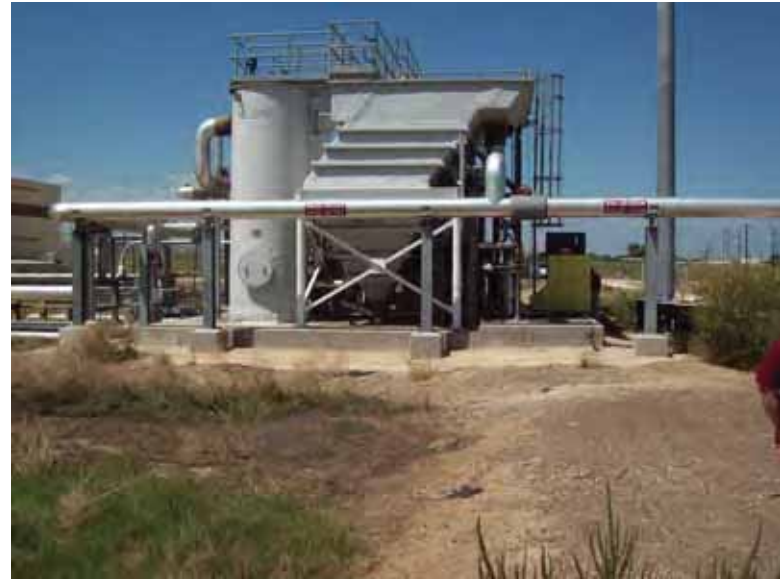
Photo 78: SP - SRH Pond clarifier structure at west embankment crest, looking north.
