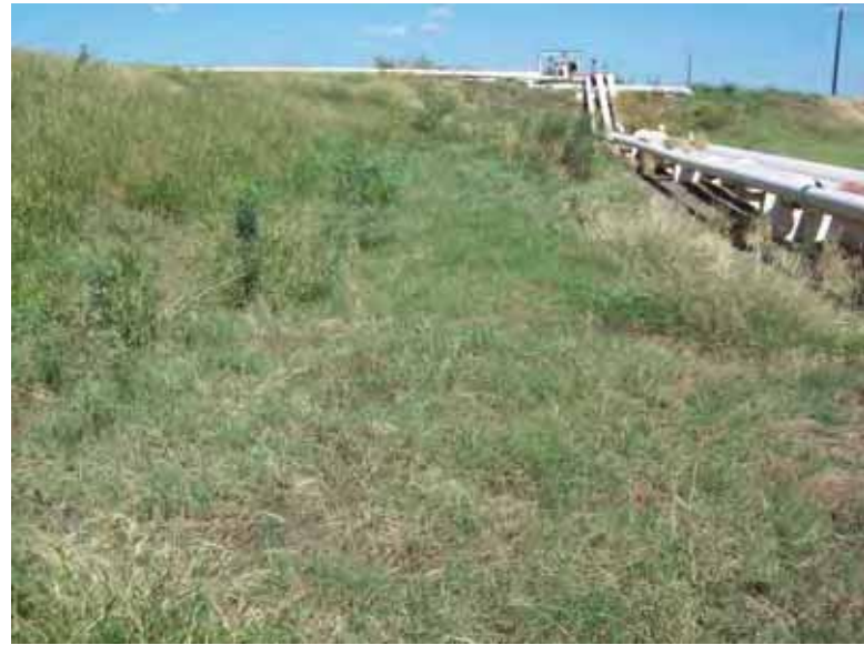
Photo 54: South embankment exterior slope, looking east.
