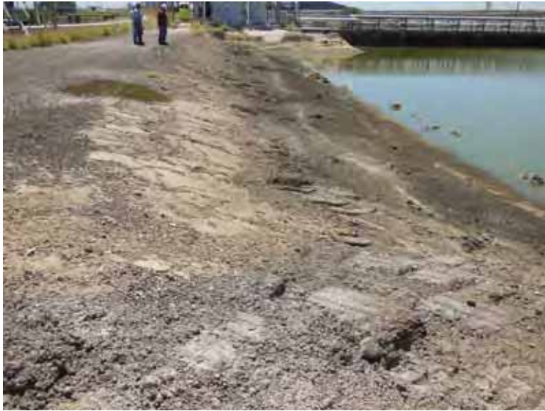
Photo 37: NP - West embankment exterior slope, looking south.
