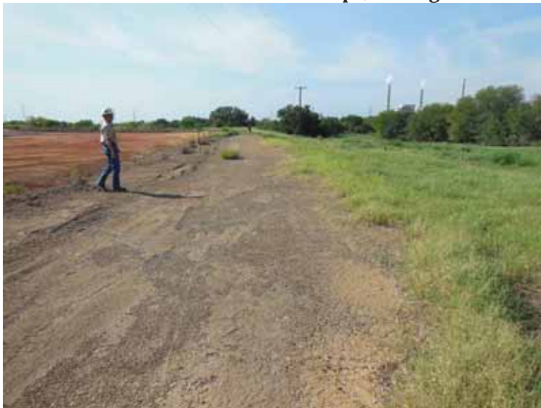
Photo 76: West embankment crest, looking south.
