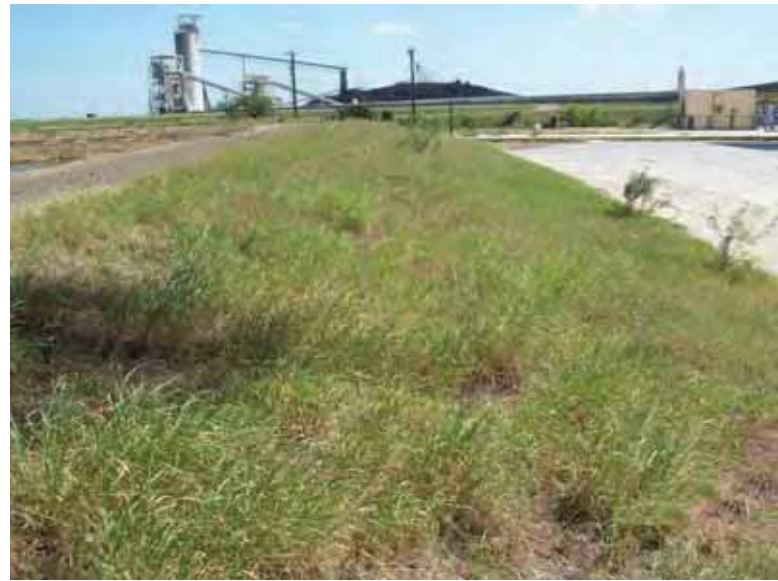
Photo 46: West embankment exterior slope, looking south.
