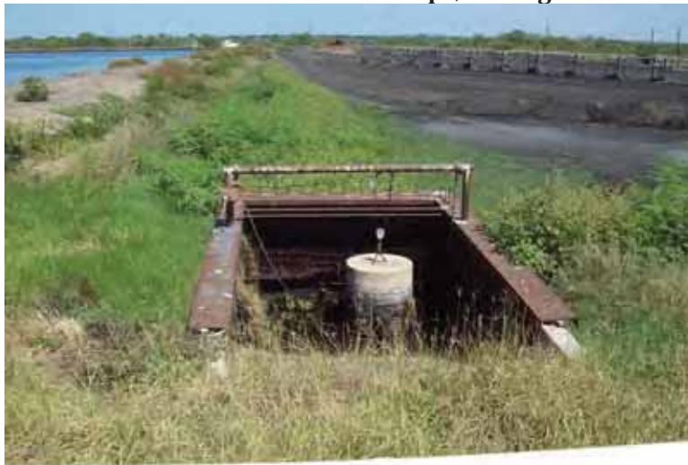
Photo 81: SP - Spillway between SRH Pond and South Bottom Ash Pond at west embankment exterior slope, looking west.
