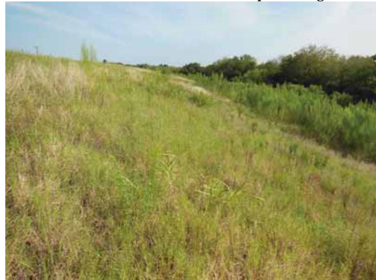
Photo 61: East embankment exterior slope, looking north.
