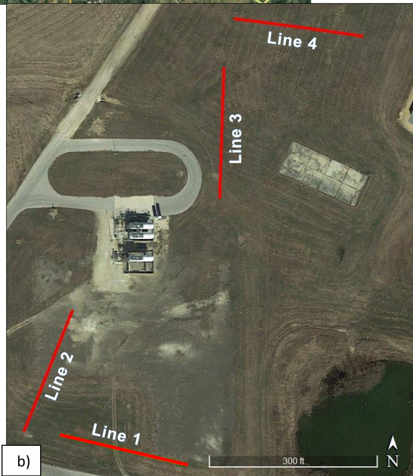
Figure 1. A) Approximate site location indicated by red star; b) line locations indicated by red lines.
