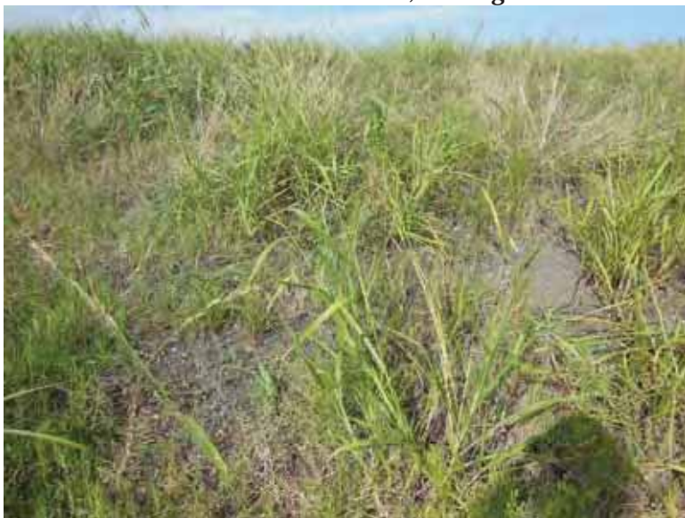
Photo 92: Loose soils on east embankment exterior slope.
