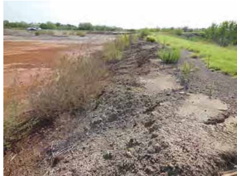
Photo 115: South embankment interior slope, looking east.
