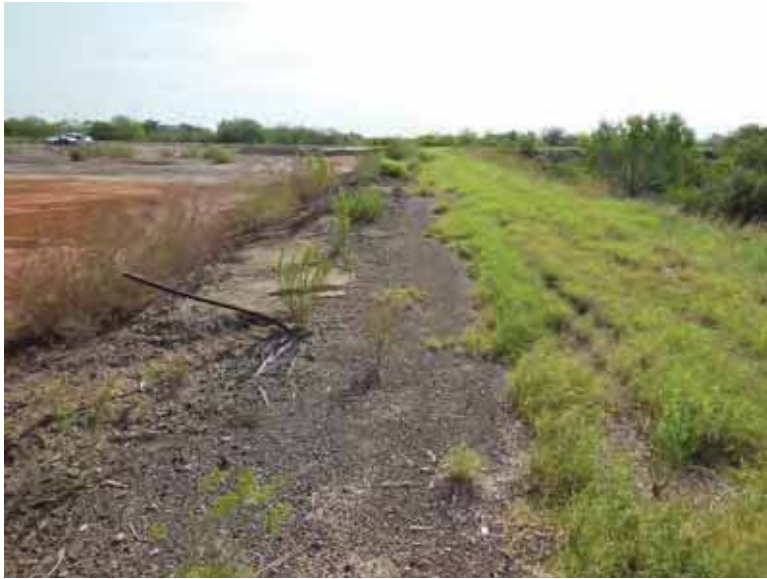
Photo 82: South embankment crest, looking east.
