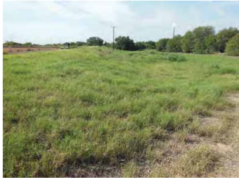
Photo 107: West embankment exterior slope, looking south.
