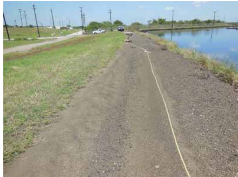
Photo 42: NP - West embankment crest, looking northeast.
