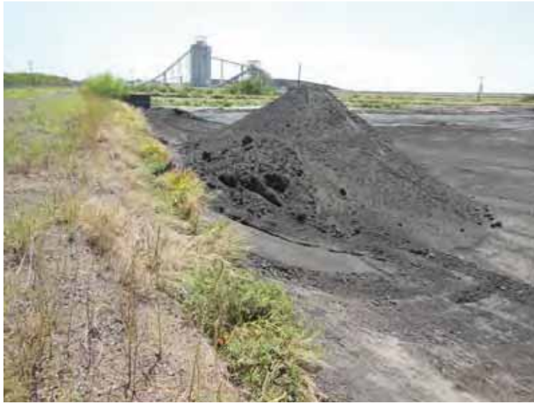
Photo 57: SP - Ash/soil pile on east embankment interior slope, looking south.
