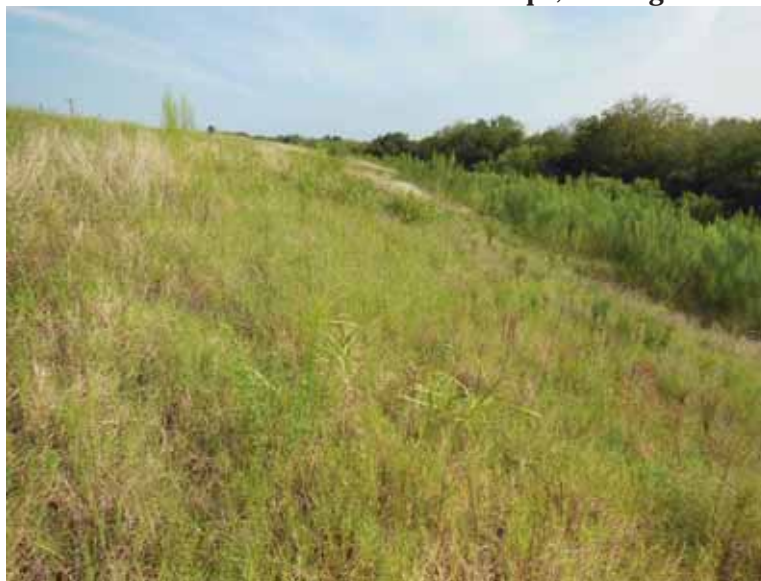
Photo 93: East embankment exterior slope, looking north.
