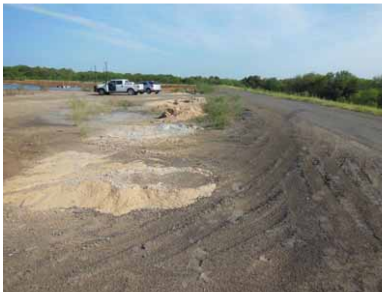
Photo 91: East embankment interior slope, looking north.
