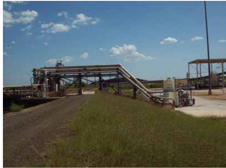
Photo 22: West embankment exterior slope, looking south.
