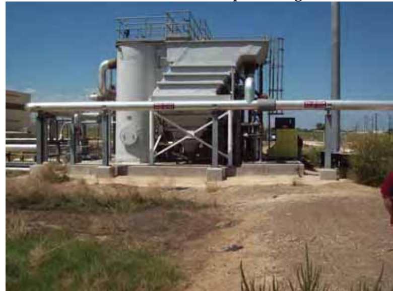
Photo 8: SRH Pond clarifier structure at east embankment crest, looking north.
