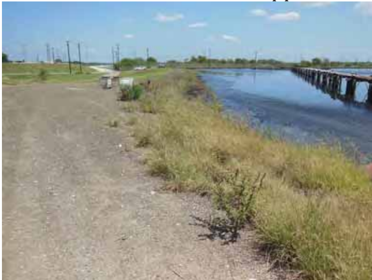
Photo 35: NP - West embankment interior slope, looking northeast.
