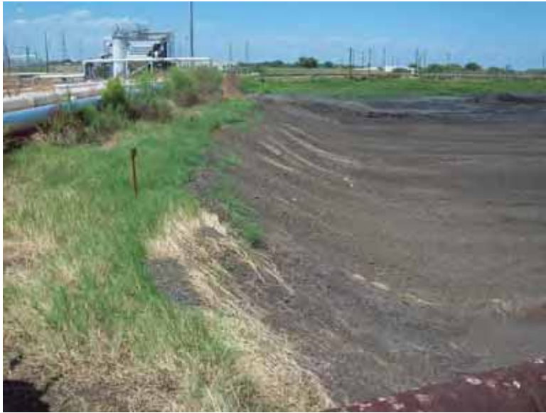
Photo 1: East embankment interior slope, looking north.
