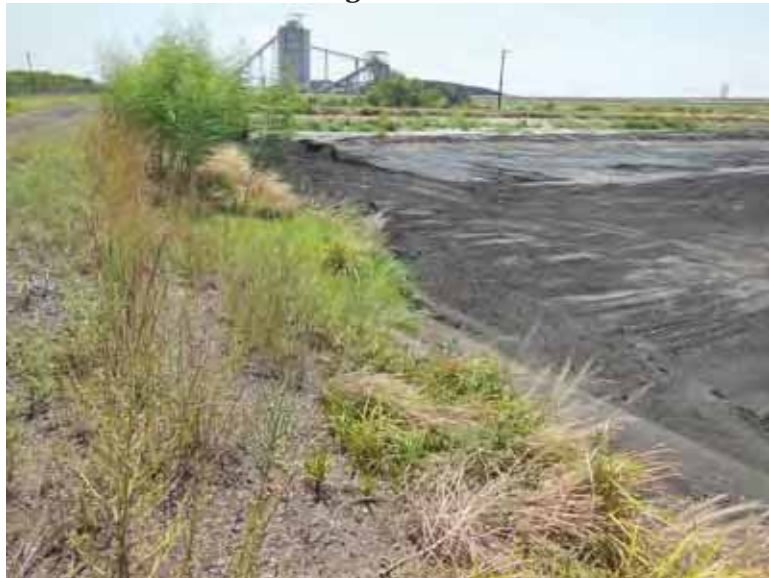
Photo 59: SP - East embankment interior slope, looking south.
