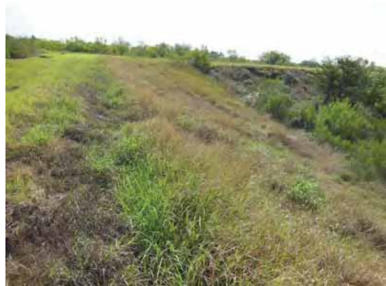
Photo 121: South embankment exterior slope, looking east.
