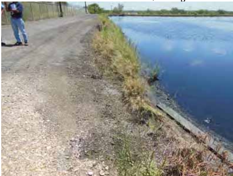
Photo 3: NP - North embankment interior slope, looking east.
