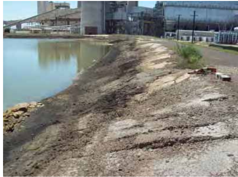
Photo 14: North embankment interior slope, looking west.
