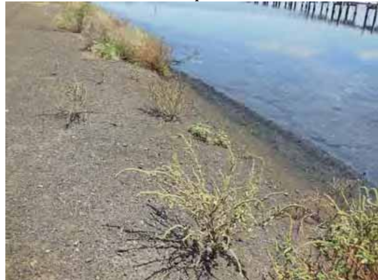
Photo 40: NP - West embankment interior slope, looking northeast.
