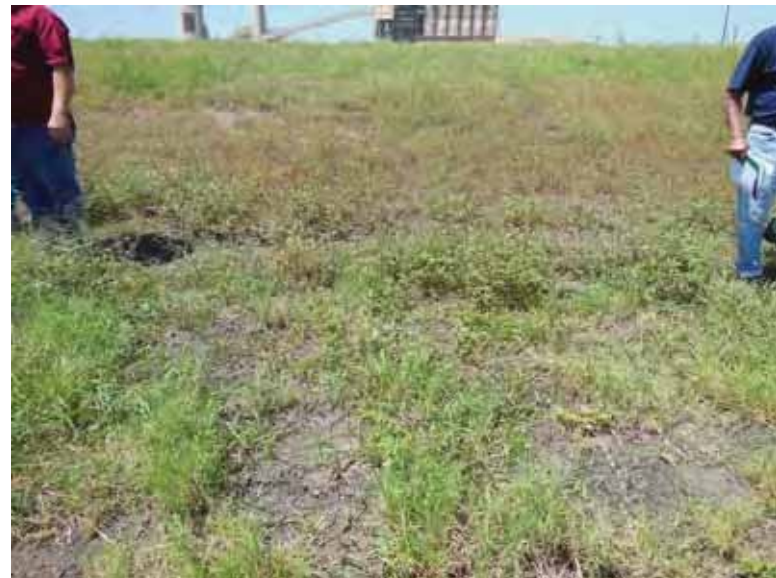
Photo 16: NP - East embankment exterior slope, looking west.
