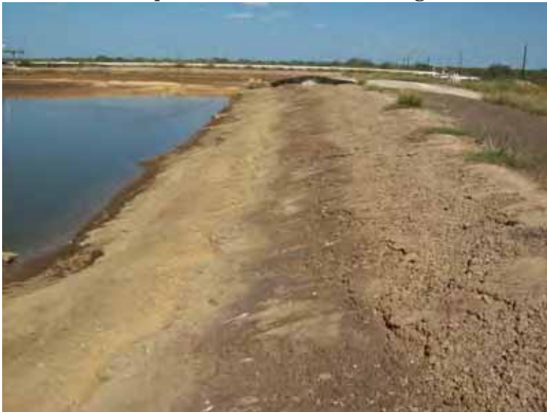
Photo 51: South embankment interior slope, looking east.
