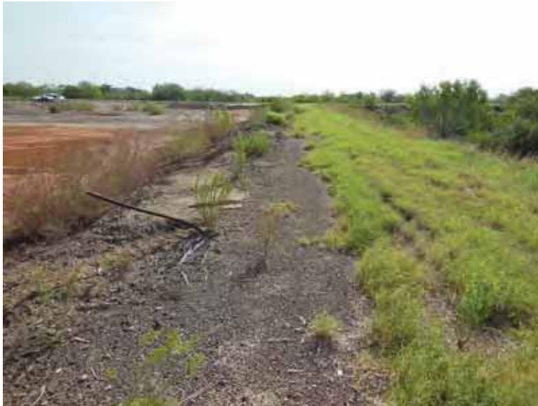
Photo 114: South embankment crest, looking east.
