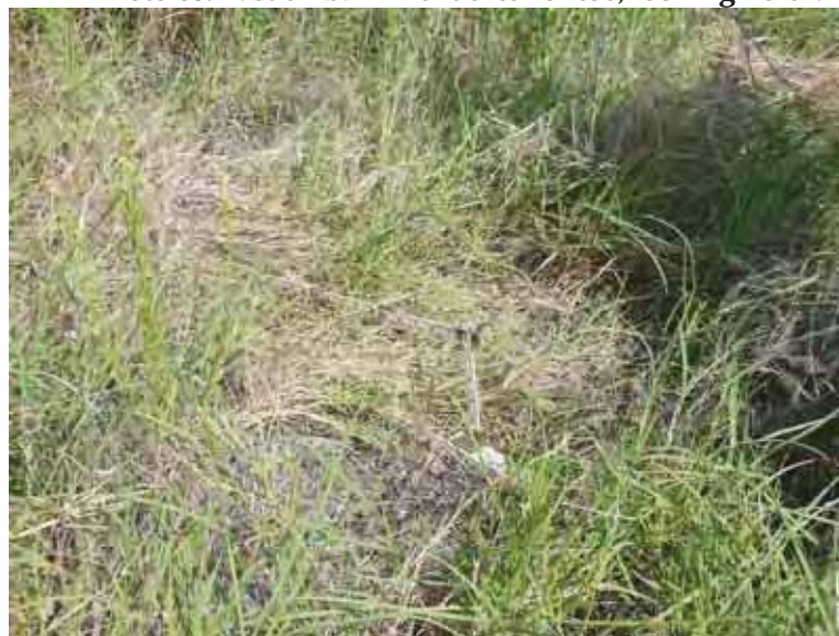
Photo 65: East embankment exterior slope measured approximately 4H:1V.
