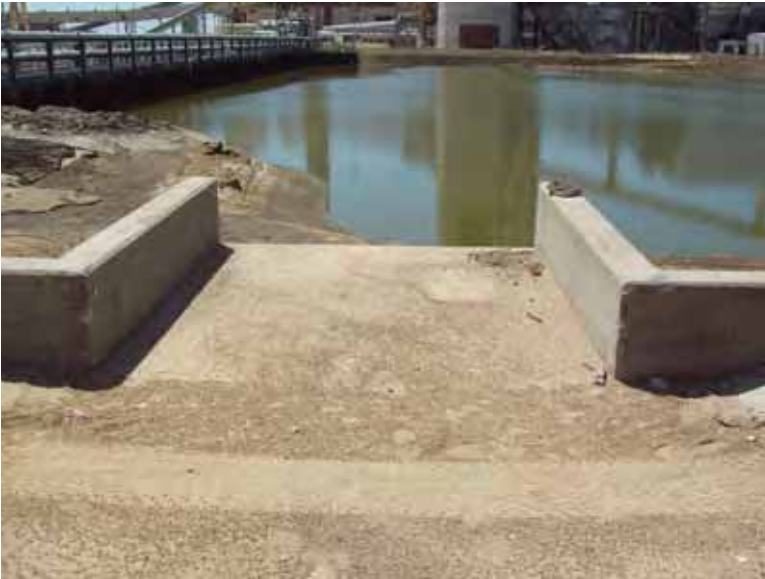
Photo 81: SP - Spillway between SRH Pond and South Bottom Ash Pond at west embankment exterior slope, looking west.
