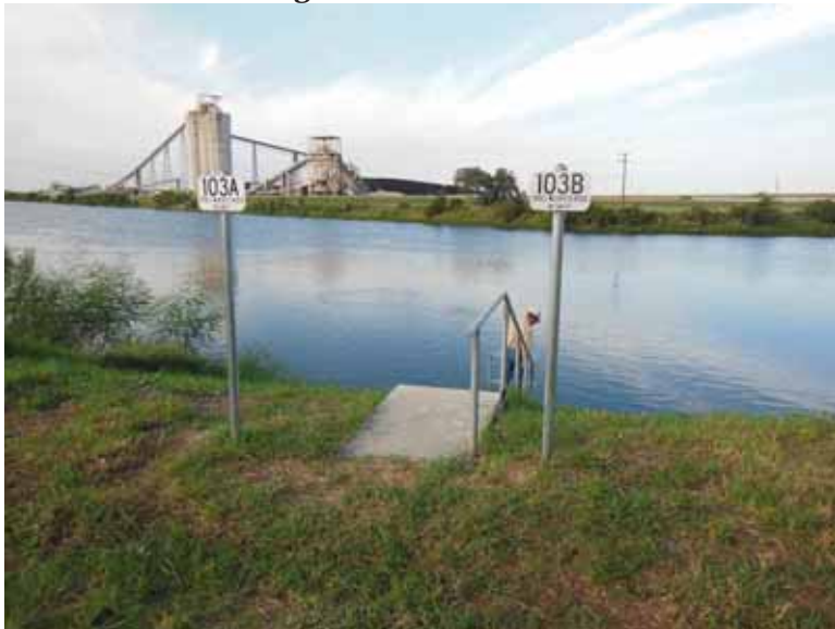
Photo 87: NP/SP - Discharge outfalls 103A and 103B into Plant intake canal.
