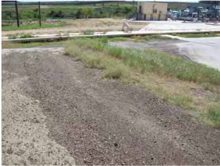
Photo 49: Exterior slope at southwest corner, looking southwest.
