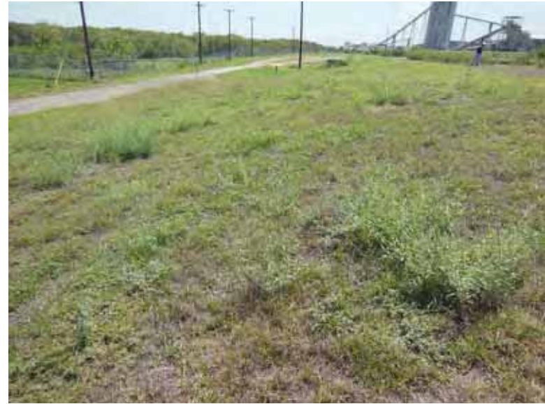
Photo 58: SP - East embankment exterior slope, looking south.
