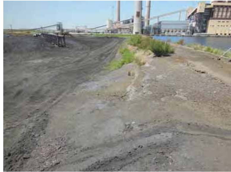
Photo 22: NP/SP - Common embankment south slope, looking west.
