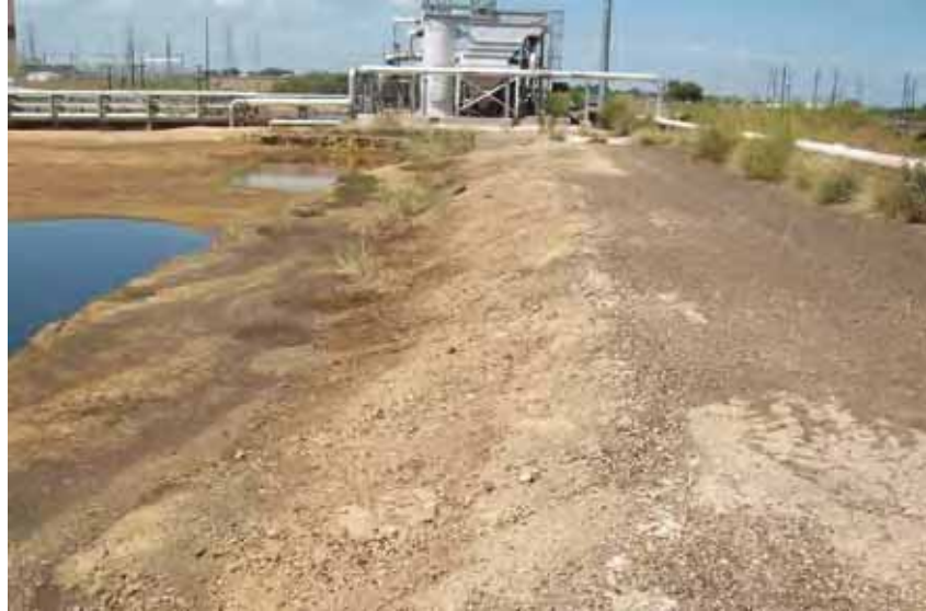
Photo 74: SP - West embankment exterior slope, looking north.
