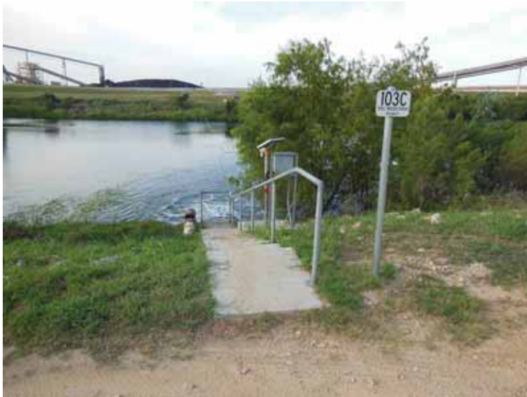
Photo 85: NP/SP - Discharge outfall 103C into Plant intake canal.
