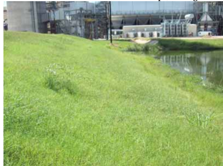
Photo 16: North embankment exterior slope, looking west.
