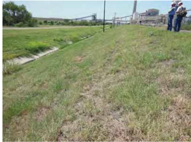
Photo 62: SP - South embankment exterior slope, looking west.
