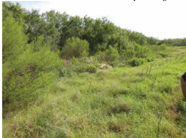
Photo 73: Trees at north embankment exterior toe, looking east.
