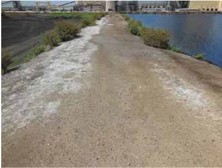
Photo 29: NP/SP - Common embankment crest, looking west.
