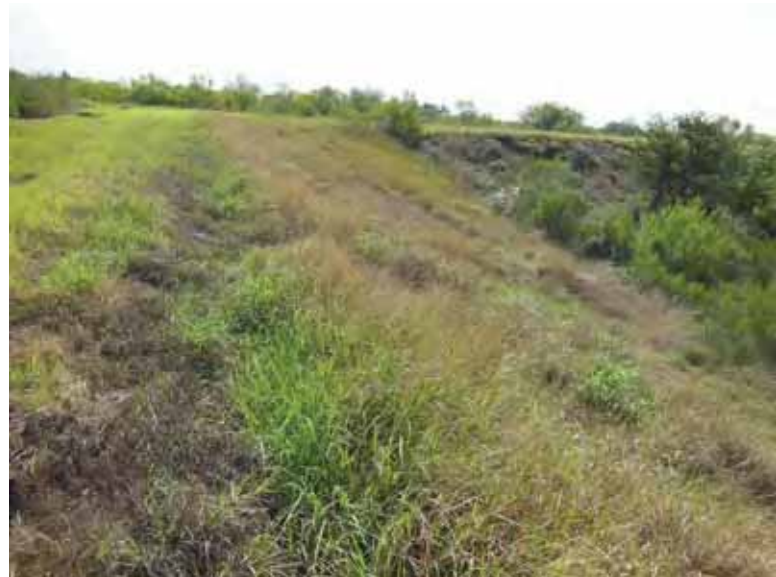
Photo 89: South embankment exterior slope, looking east.
