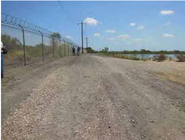
Photo 1: NP - North Embankment crest, looking east.
