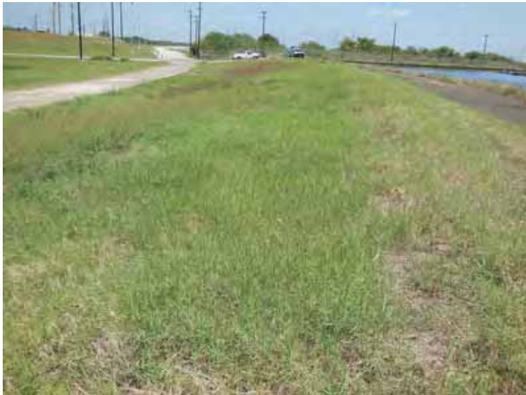
Photo 39: NP - West embankment exterior slope, looking northeast.
