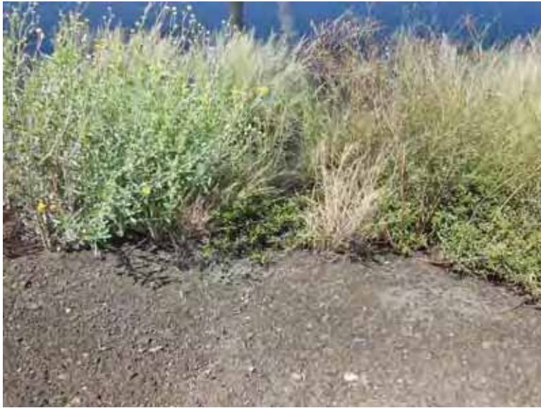
Photo 13: NP - East embankment interior slope, looking west. Note vegetation on slope.
