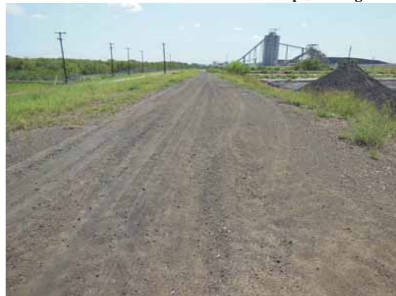
Photo 56: SP - East embankment crest, looking south.
