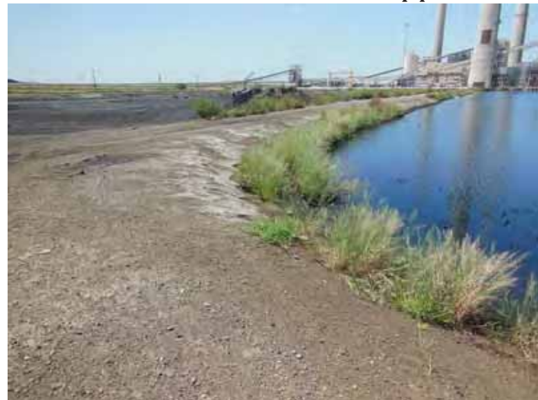
Photo 20: NP - Interior slope at southeast corner, looking west.
