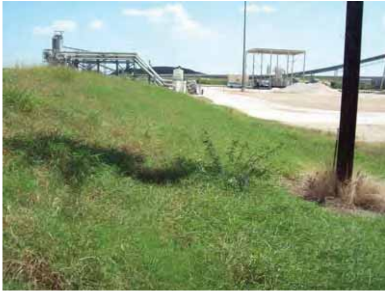
Photo 21: West embankment exterior slope, looking south.
