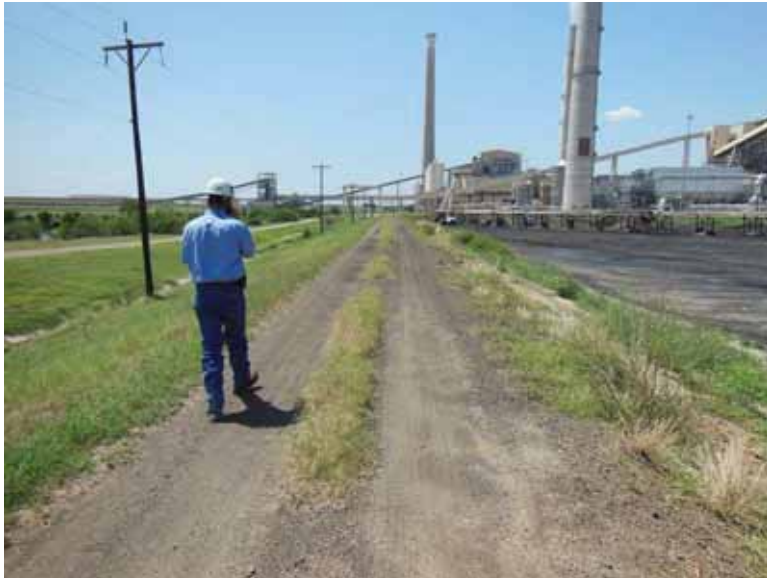
Photo 65: SP – South embankment crest, looking west.
