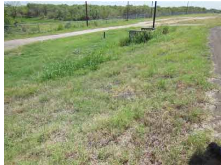
Photo 60: SP - Exterior slope at southeast corner, looking south.
