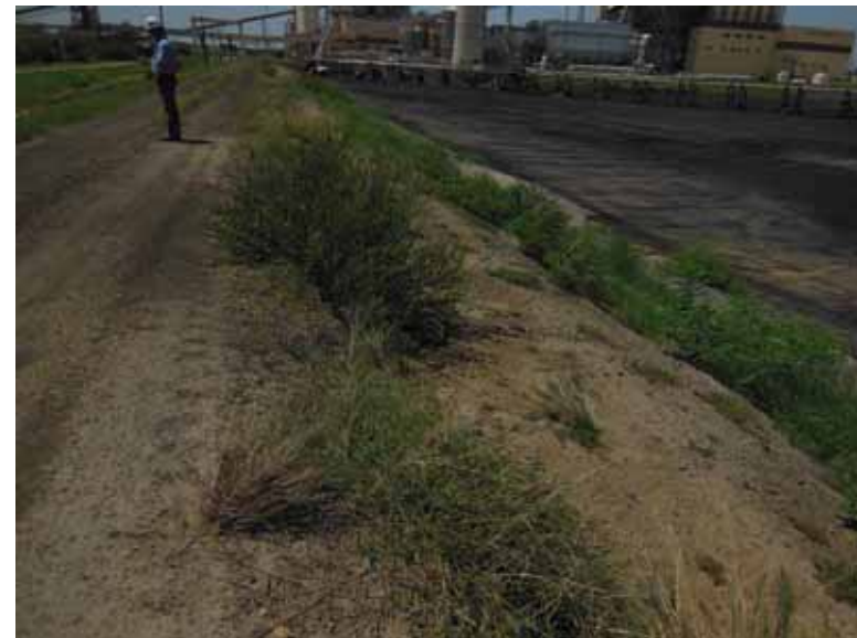
Photo 64: SP - South embankment interior slope, looking west.
