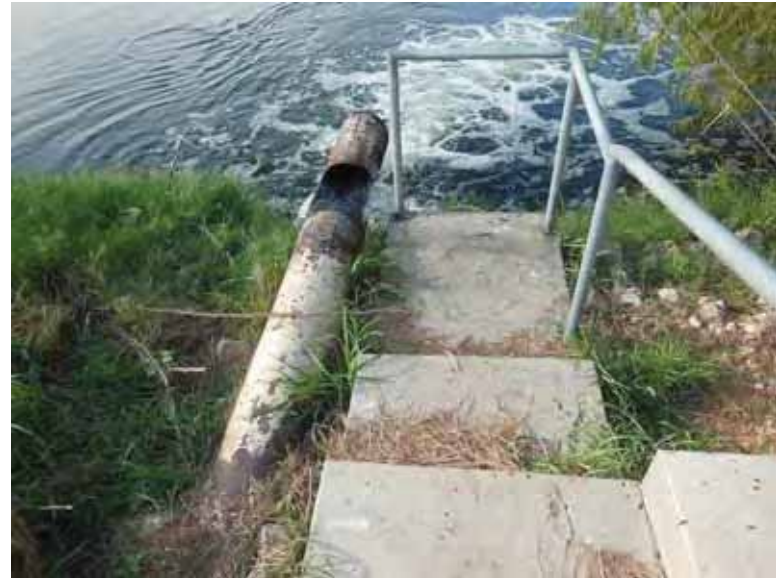
Photo 86: NP/SP - 12-inch-diameter piping at outfall 103C.
