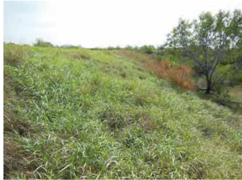
Photo 119: South embankment exterior slope, looking east.
