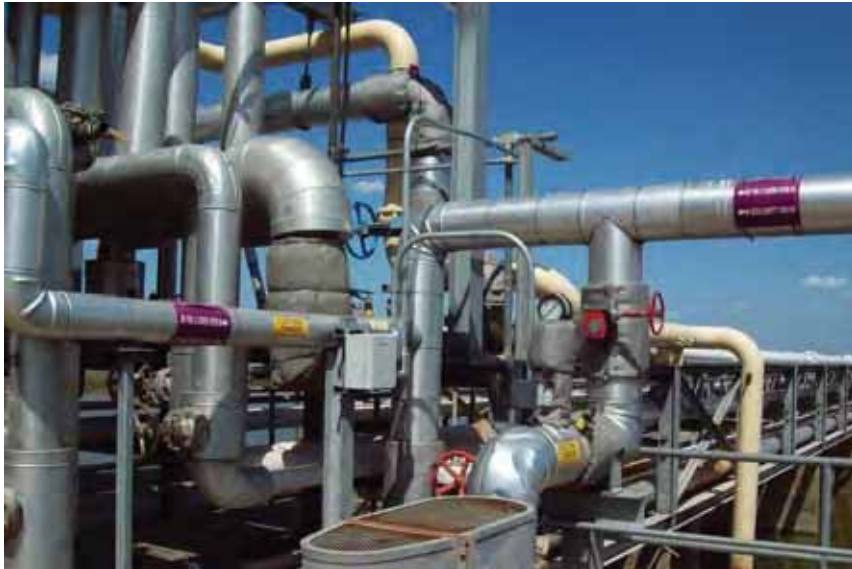
Photo 25: Piping at west embankment interior slope, looking northeast.
