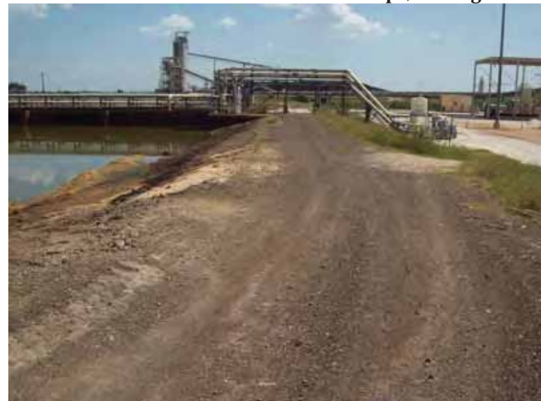
Photo 20: East embankment crest, looking south.
