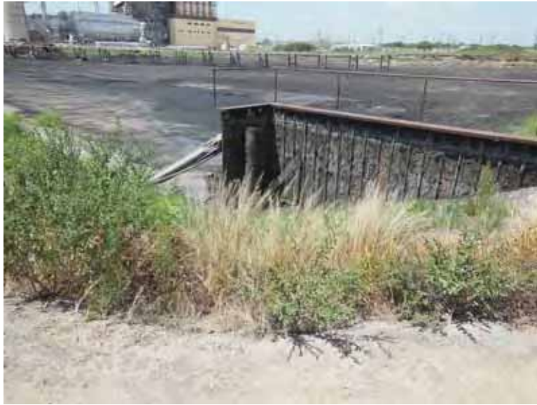
Photo 61: SP - Outlet structure at southeast corner interior slope, looking northwest.
