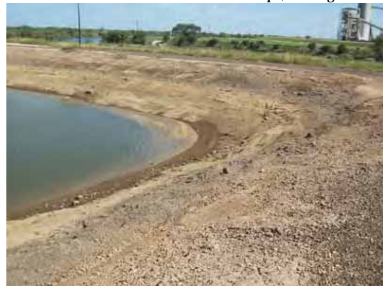
Photo 48: Interior slope at southwest corner interior slope, looking southeast.
