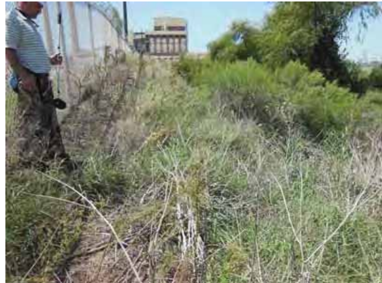
Photo 48: NP - North embankment exterior slope, looking west.
