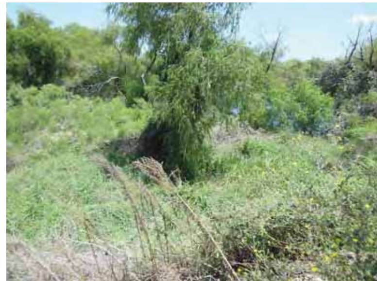
Photo 8: NP - North embankment exterior slope, looking north. Calaveras Lake in distance.
