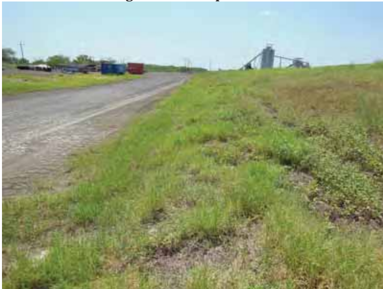
Photo 15: NP - East embankment exterior slope, looking south.
