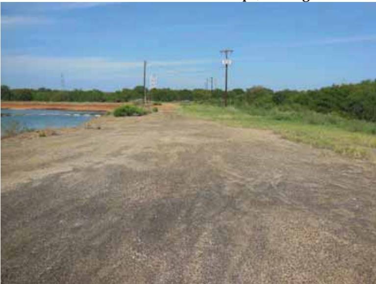
Photo 100: North embankment crest, looking west.
