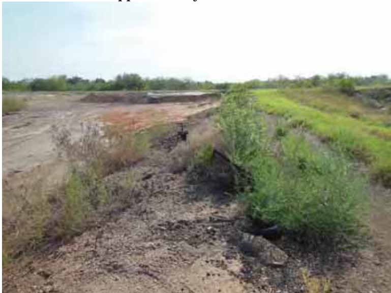
Photo 120: South embankment interior slope, looking east.
