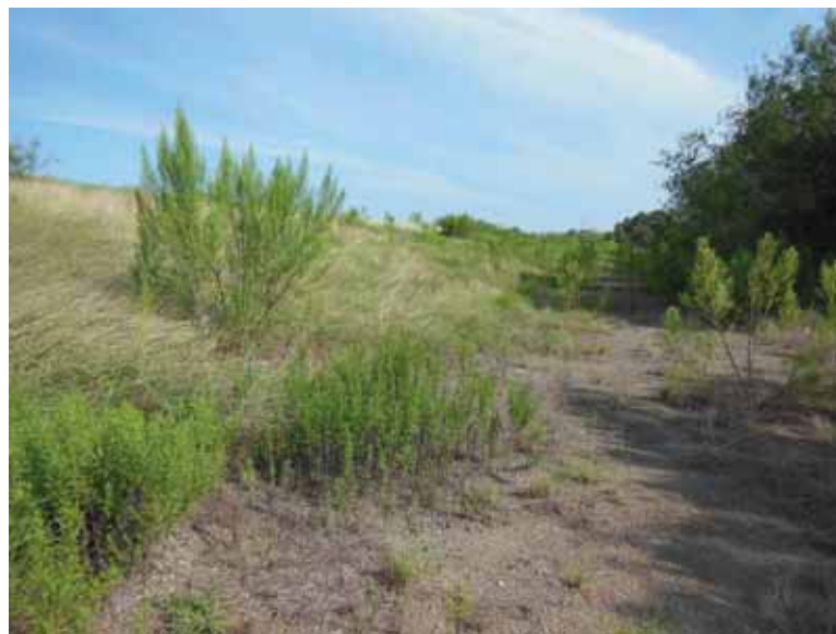
Photo 63: East embankment exterior toe, looking north.
