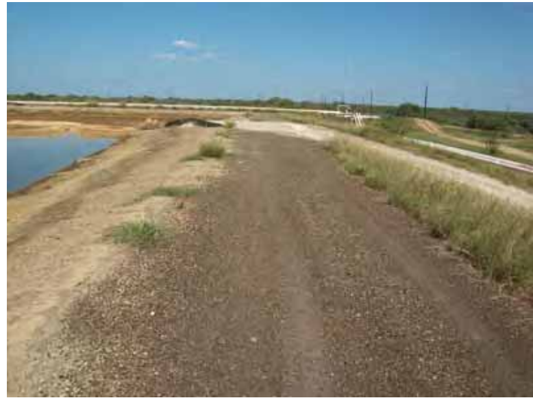
Photo 50: South embankment crest, looking east.
