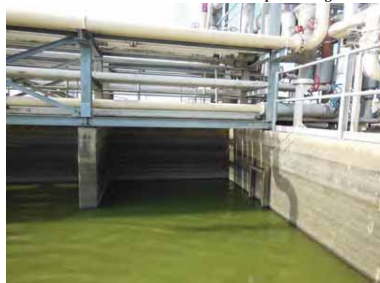
Photo 24: Submerged SRH-north outlet structure at west embankment interior slope, looking south.
