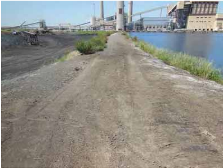
Photo 21: NP/SP - Common embankment crest, looking west.
