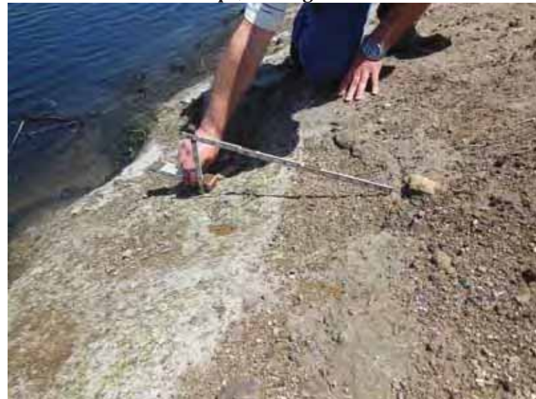
Photo 28: NP/SP - Common embankment north slope, looking east. Slope measured approximately 3H:1V.
