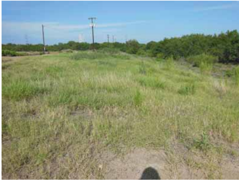
Photo 98: North embankment exterior slope, looking west.
