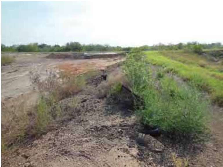
Photo 88: South embankment interior slope, looking east.
