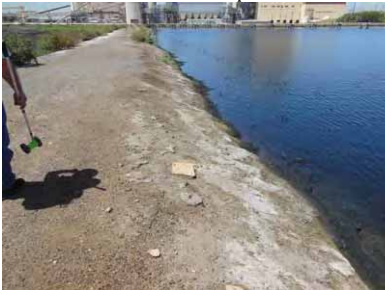
Photo 27: NP/SP - Common embankment north slope, looking west.
