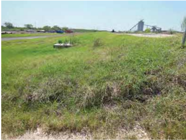
Photo 9: NP - East embankment exterior slope, looking south.
