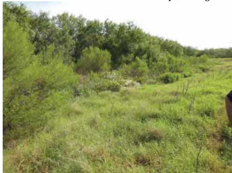
Photo 105: Trees at north embankment exterior toe, looking east.
