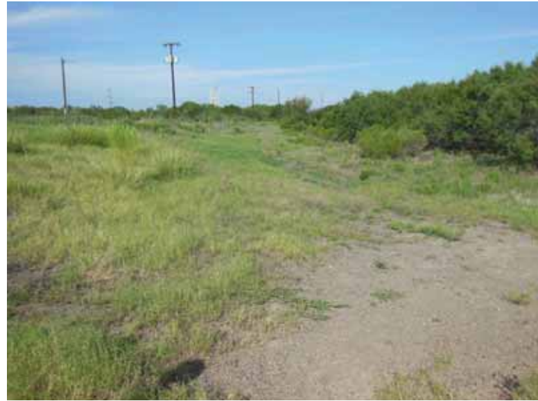
Photo 99: North embankment exterior slope, looking west.
