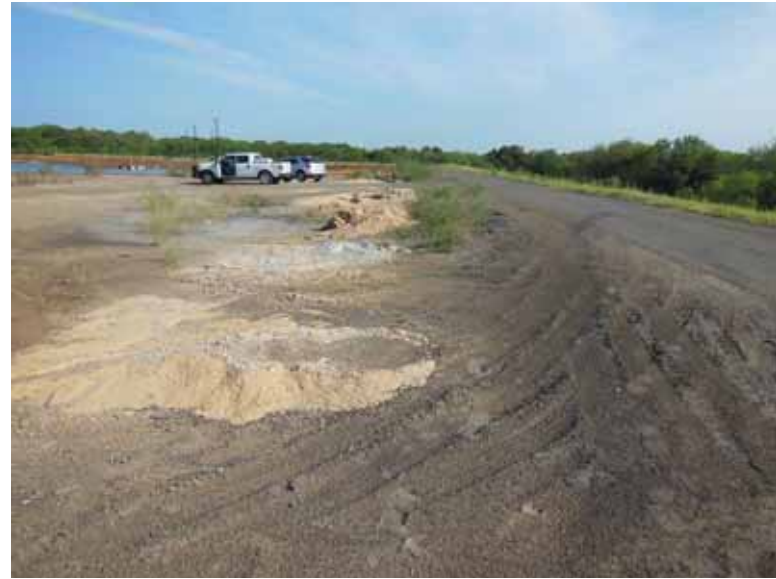
Photo 59: East embankment interior slope, looking north.
