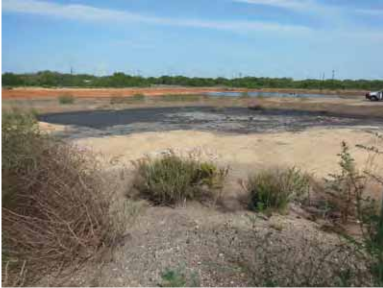
Photo 90: Interior slope at southeast corner, looking northwest.
