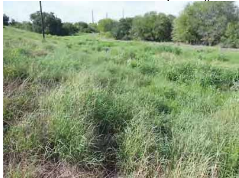
Photo 109: West embankment exterior slope, looking southwest.
