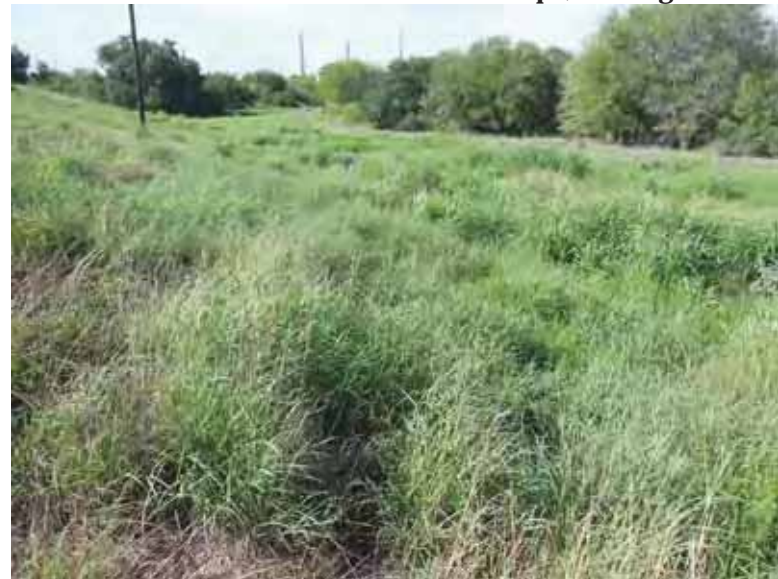
Photo 77: West embankment exterior slope, looking southwest.
