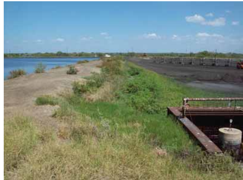
Photo 84: NP/SP - Common embankment south slope, looking east.
