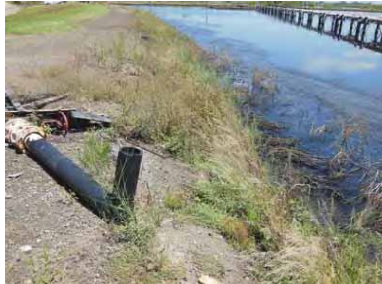
Photo 36: NP - North embankment interior slope, looking northeast.
