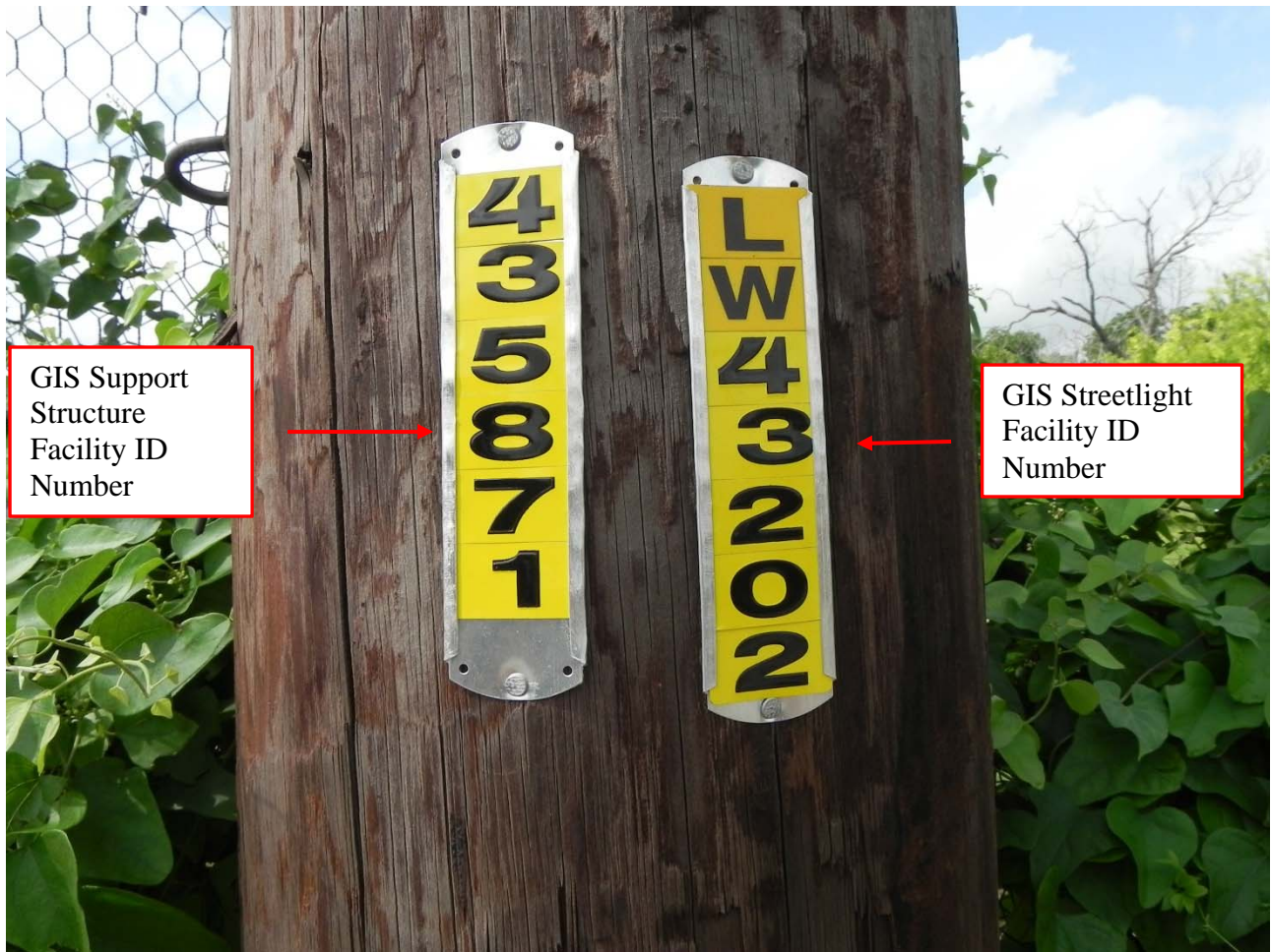
Figure 9 Photo of Pole with Support Structure and Streetlight Number Applied
