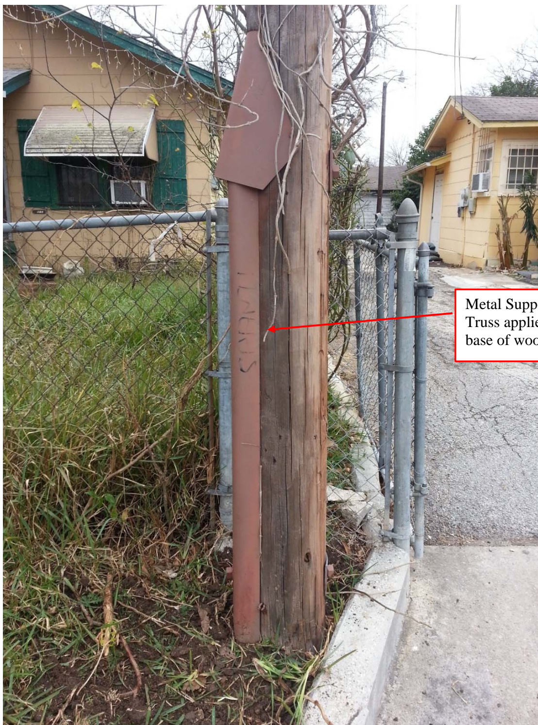
Figure 10 Pole with Steel Truss Installed
