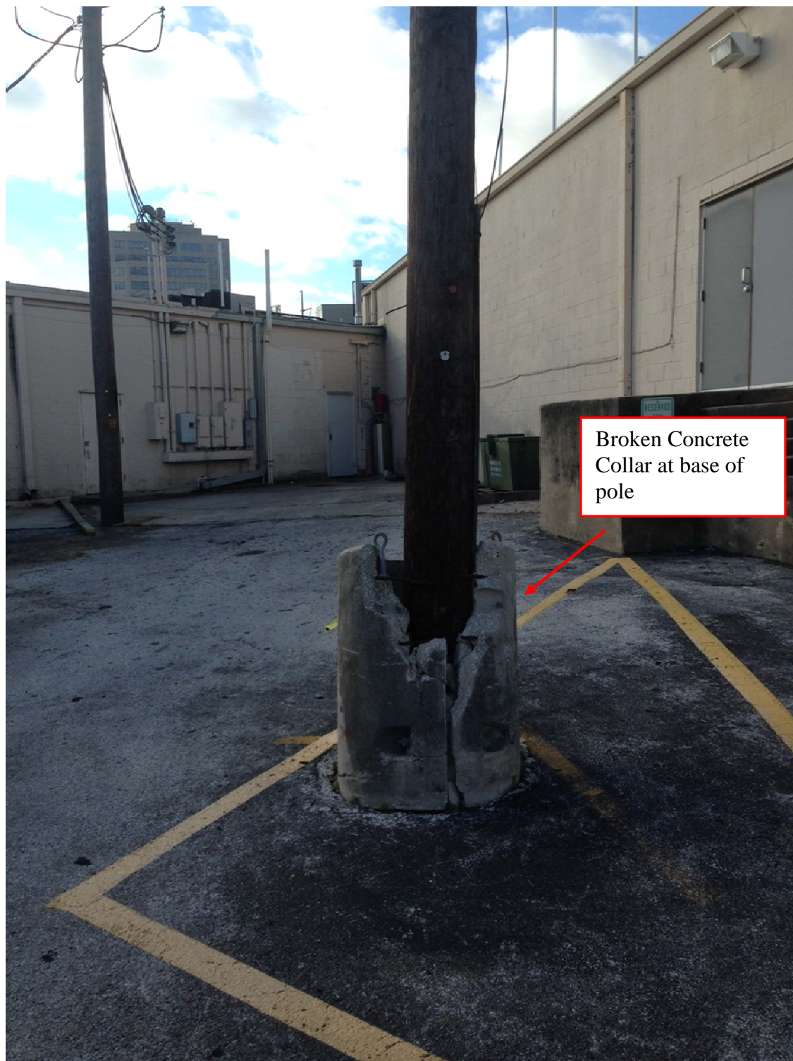
Figure 17 Pole with Concrete Collar at Base
