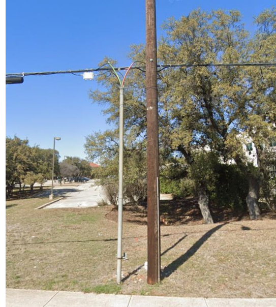
Stand off bracket not attached
