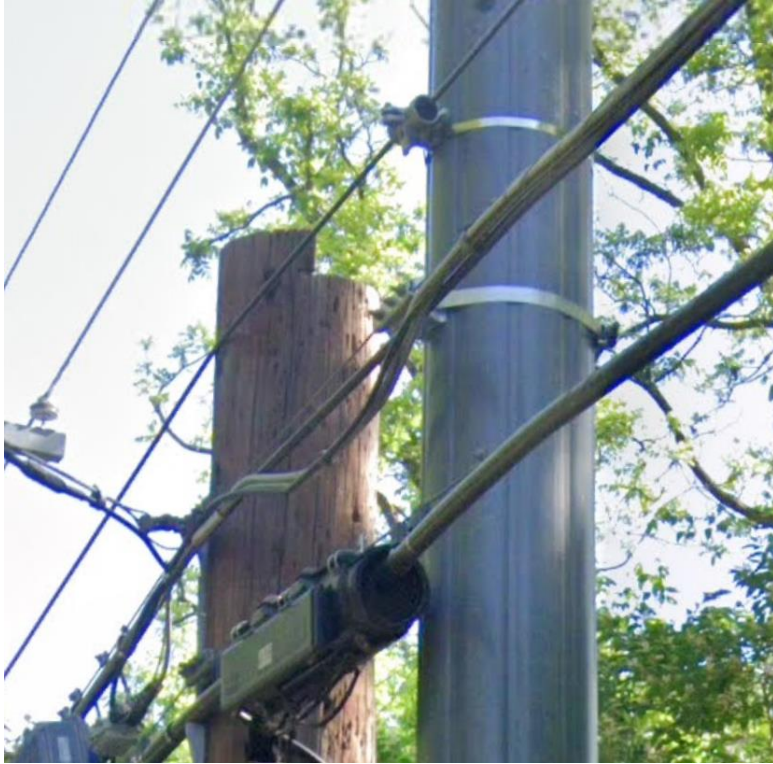
Field Application of Banding Kits
