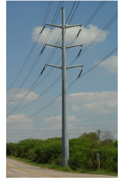
Steel Pole Structure
