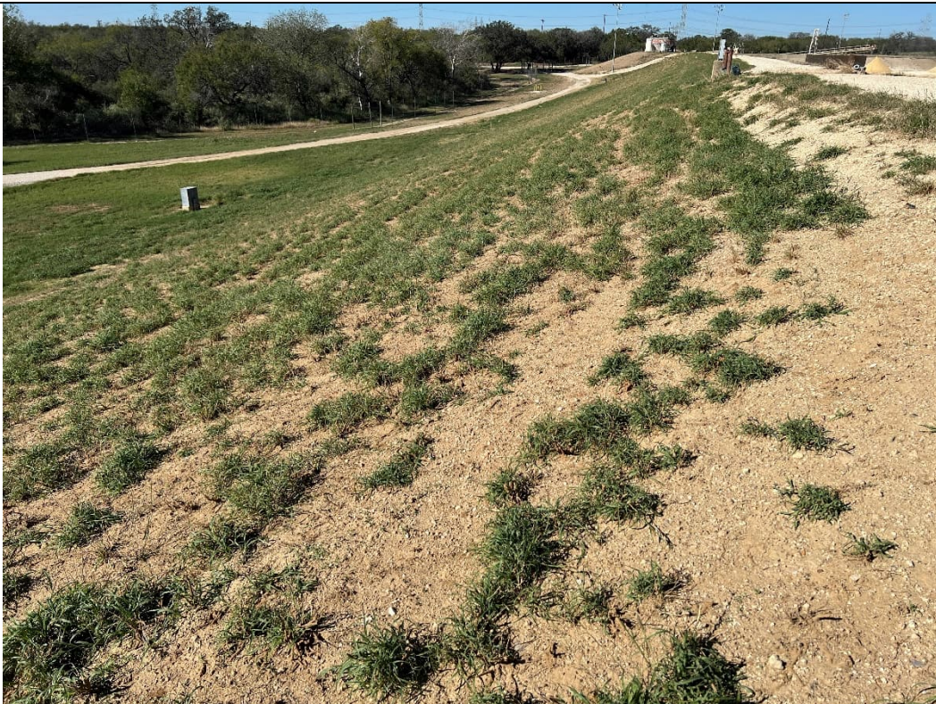
Photograph: 10 Fly Ash Landfill – standing on south berm – facing west. Some bare spots noted – no significant erosion. Photo taken 11/10/2025.
