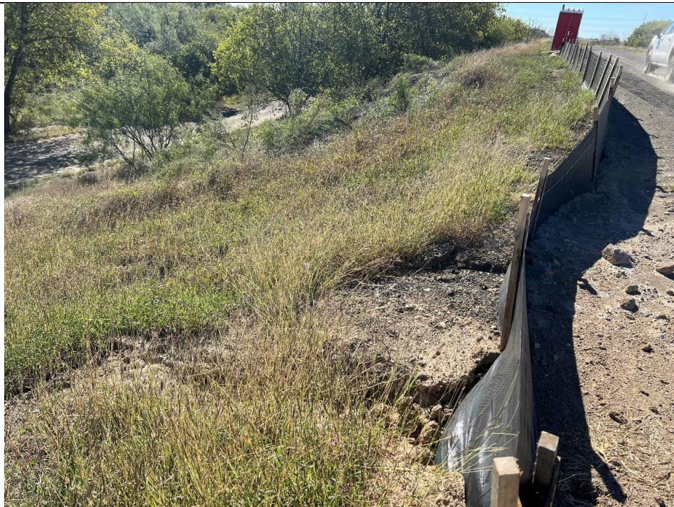
Photograph: 18 Evaporation Pond – standing on east berm – facing south. Some erosion noted at exterior top of berm and silt fence. Photo taken 11/10/2025.
