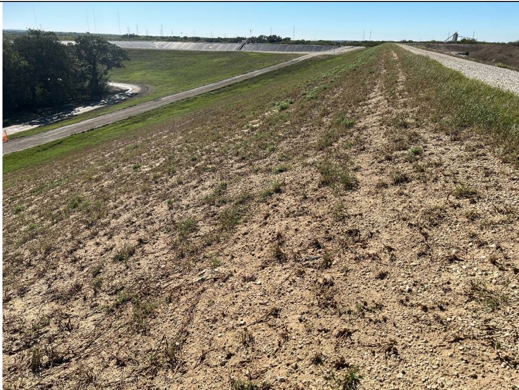
Photograph: 6 Fly Ash Landfill – standing on northeast corner – facing south. Some bare spots noted – no significant erosion. Photo taken 11/10/2025.
