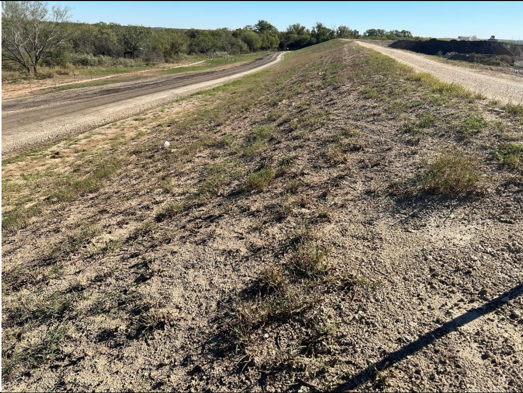
Photograph: 1 Fly Ash Landfill – standing on west berm – facing north. Some bare spots noted – no significant erosion. Photo taken 11/10/2025.
