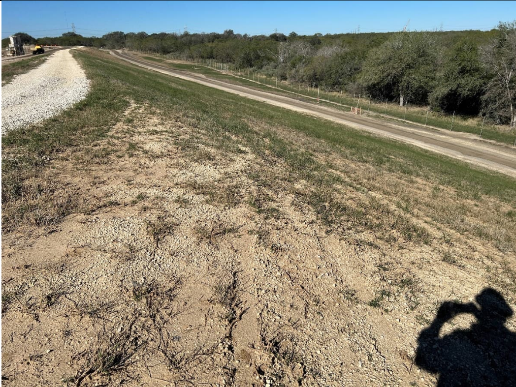
Photograph: 3 Fly Ash Landfill – standing on northeast corner – facing west. Some bare spots noted – no significant erosion. Photo taken 11/10/2025.
