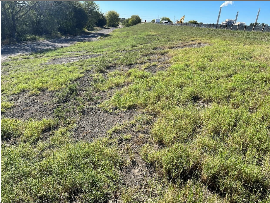
Photograph: 13 Evaporation Pond – standing on northeast corner – facing south. Some bare spots noted – no significant erosion. Photo taken 11/10/2025.
