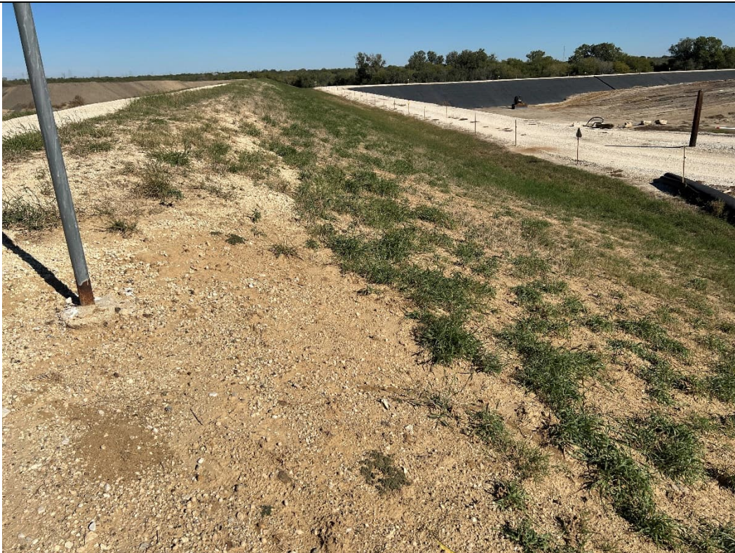
Photograph: 8 Fly Ash Landfill – standing on east berm – facing north. Some bare spots noted – no significant erosion. Photo taken 11/10/2025.
