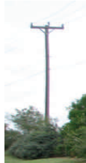
Typical Distribution Line
