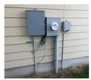
**Typical Underground Meter Loop**
