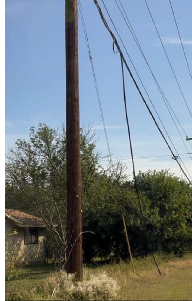
Telecommunication Wire Down
