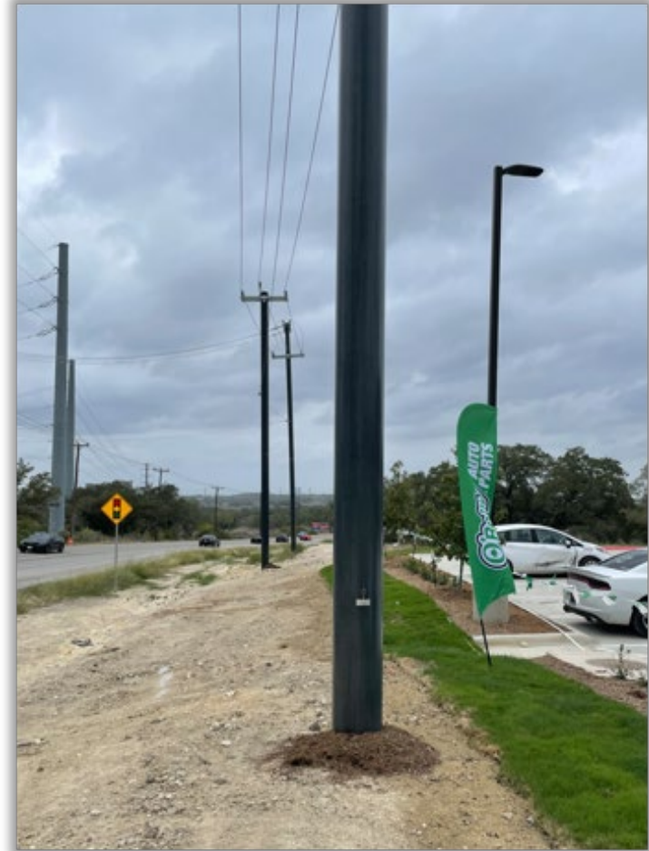
Installed Composite Pole
