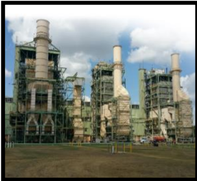
Braunig 1, 2 & 3 Gas Plant Built in 1966, 1968, 1970 859 MW
