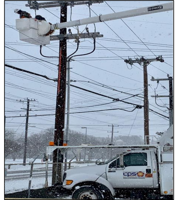
Repairs during the winter storm
