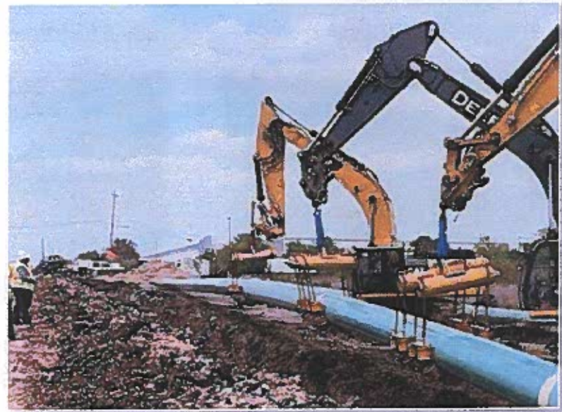
Contractor installing new supply pipe
