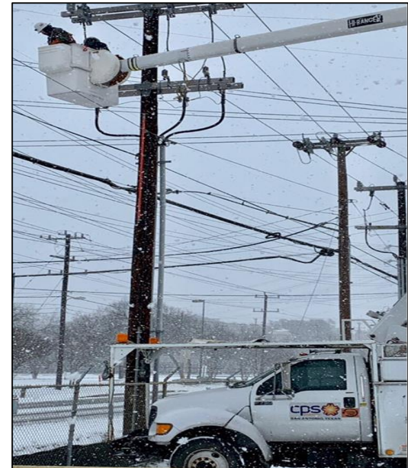
Repairs being made during Winter Storm Uri
