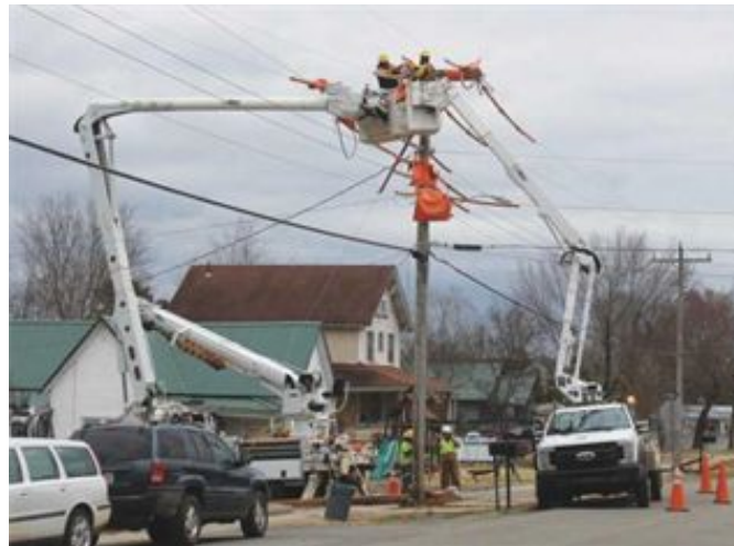
Contract crews at work on overhead distribution systems
