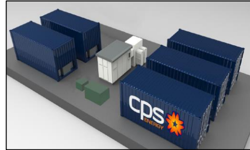
10 MW Battery Storage System
