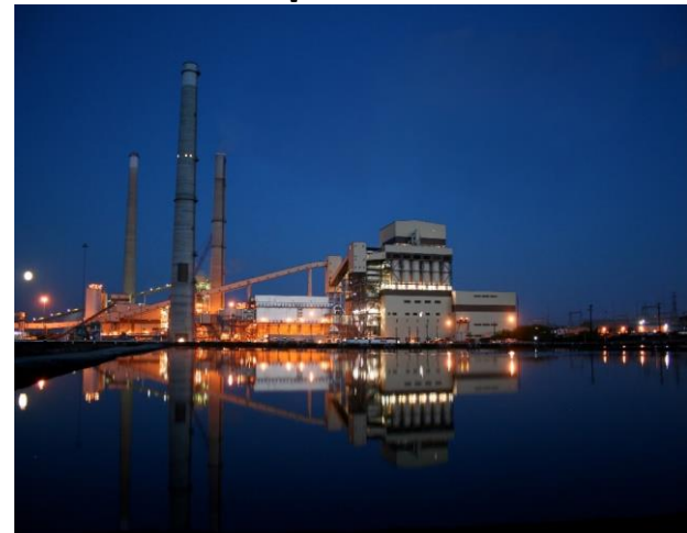
1350 MW Spruce Plant
