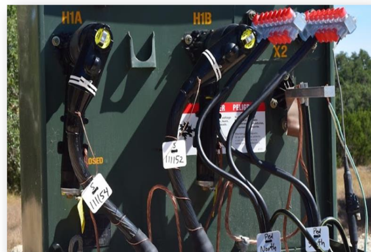
Terminated Cable for New Pad-Mount Transformer
