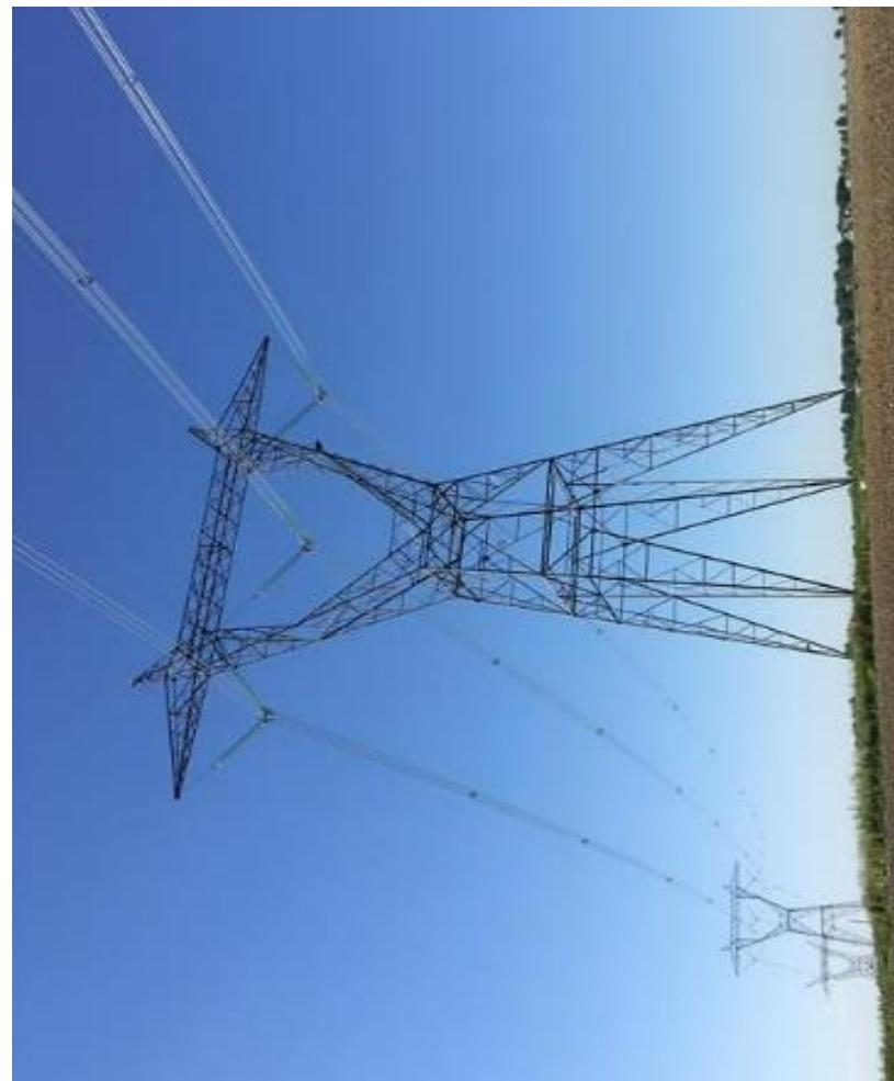
Typical 765kV Lattice Structure
