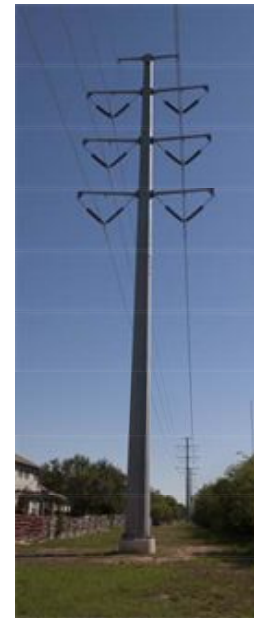
Double Circuit Transmission Pole Line
